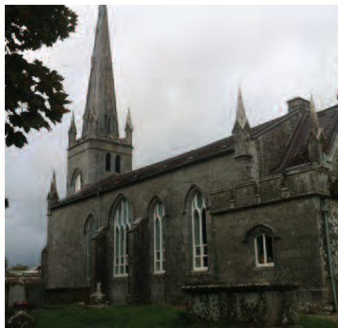
Carrigaline Church of Ireland is a handsome edifice of hewn limestone, in Neo Gothic style having a square tower crowned with pinnacles and surmounted by an elegant and lofty octagonal spire. The Church was erected in 1823, near the site of the former church, and enlarged in 1835.
