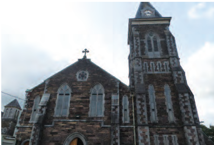
St. Coleman's RC Church, Macroom, built in 1841 and remodelled and enlarged in 1893 to the design of Dominic Coakley.
