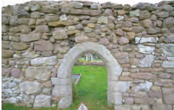
The 15th/16th century door inserted in the south wall of the nave with stone carved head above. The low pointed door with its finely dressed limestone surround stands out against the red sandstone of the earlier wall of the nave.
