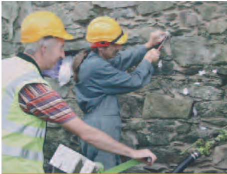
Council Conservation team repointing masonry wall of medieval church.
