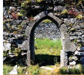
15th century limestone door surround with chamfered edge, typically located at the west end of the south wall.
