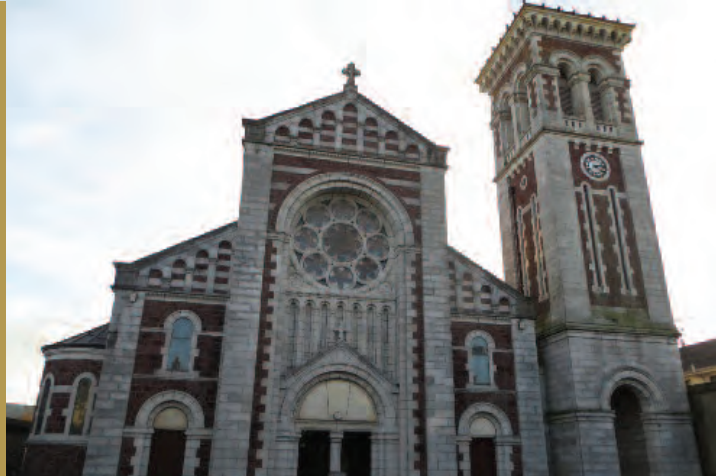
St Mary's Church, Mallow. It was built in 1818 with a T shaped plan and extended in 1900 with the addition of a dramatic Romanesque style entrance facade with loft tower, to the design of George Ashlin.
