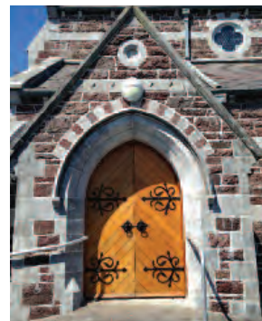
Detail of porch entrance at Sacred Heart Church in Glounthaune.
