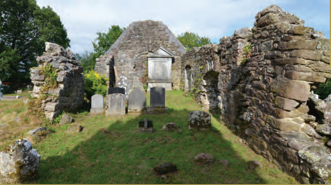
Interior of Aghacross Church, looking east into the 15th/16th century Chancel.
