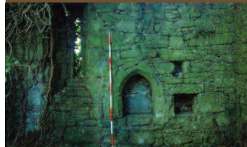
Narrow lancet window with side walls played to allow as much light in to the altar, piscina and wall press adjacent.
