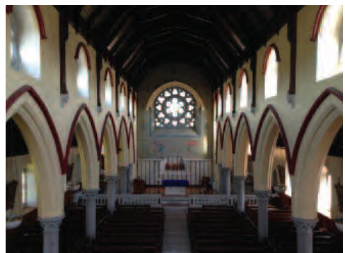
Interior of St Mary's Church, Carrigtwohill with pointed arcading opening to the side aisles and nave lit by the clerestory windows.
