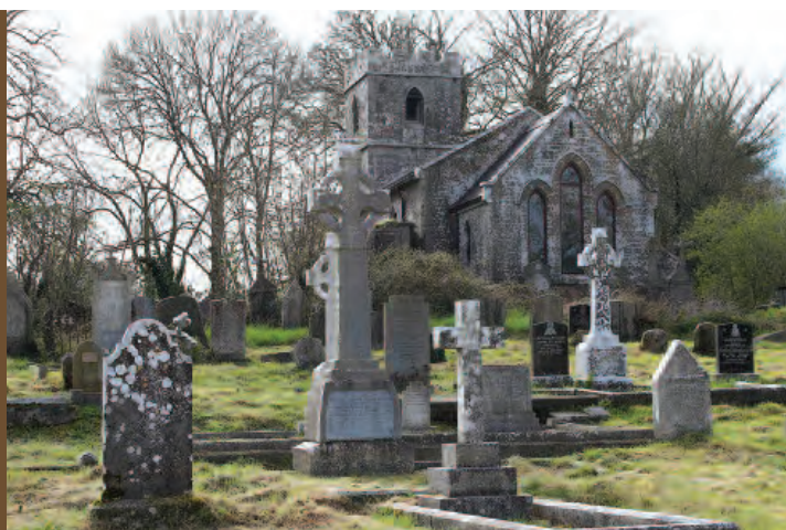
The Church of Ireland Church in Castlemagner, as viewed from the south east, was built in 1816 to accommodate 120 people on the site of the medieval parish church. The Vestry and the heating system were added in 1887 and the chancel was added in the 1900's. Image courtesy of Catherine Culloty.
