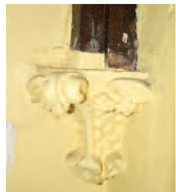
Detail of ornate plastered label stop.
