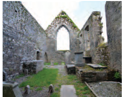
Chancel of church looking east.
