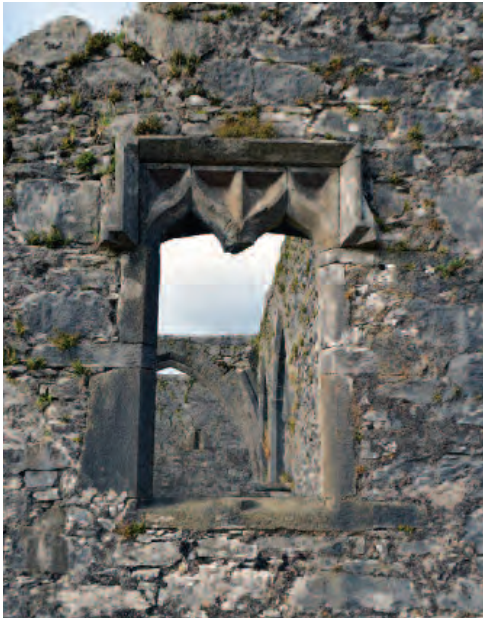
Distinctive 15th century double ogee-headed window, in south transept.
