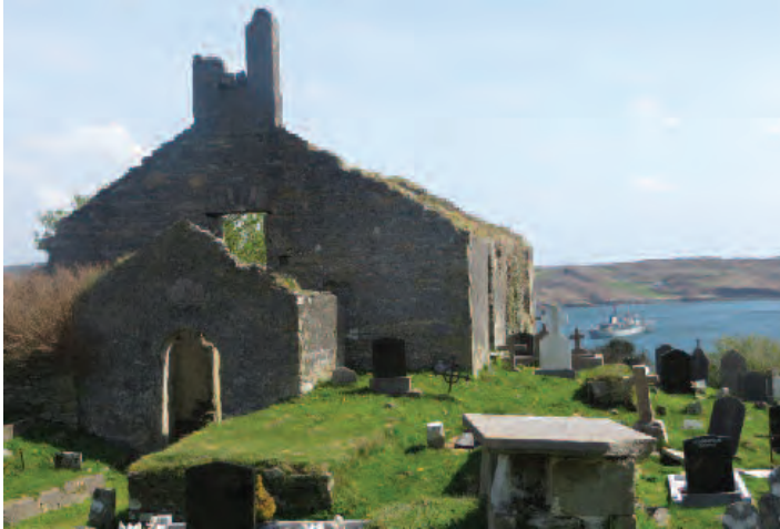
Ruins of late medieval church in Schull, which was extensively rebuilt in 1721, incorporating part of the earlier church in the north wall with its ogee headed window.
