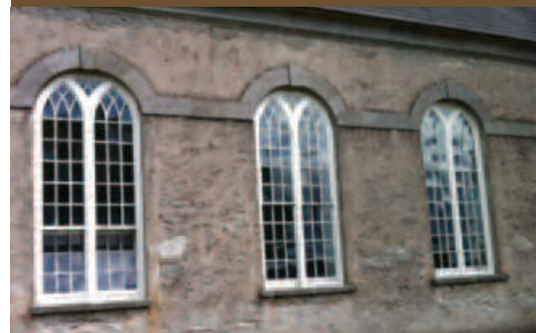
Detail of timber Y - tracery windows with delicate switch line tracery and original glass with curved cut stone cornice under eaves.
