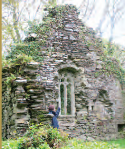
Remains of late medieval parish church of Macloneigh. Note the double round headed east window below simple tracery.
