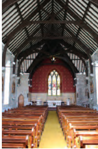
Interior of St Marys RC Church Castlemagner, built in the mid 19th century, with a very fine open timber roof supported on stone corbels.
