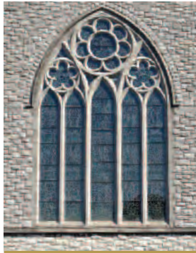
Geometric tracery window RC Church of Holy Rosary Midelton.
