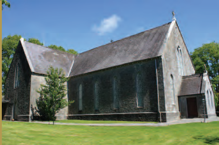
St Marys RC Church Castlemagner is an elegant example of an RC church built in 1859-60 to replace an earlier, more humble, vernacular thatched chapel. It has a very fine open timber roof supported on stone corbels.
