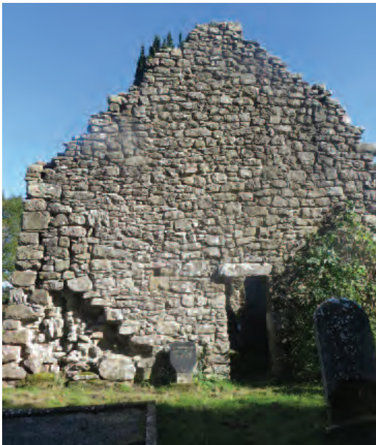
The West Gable Wall
