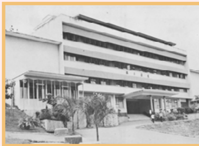
Main administration Building known as 张汉三楼
