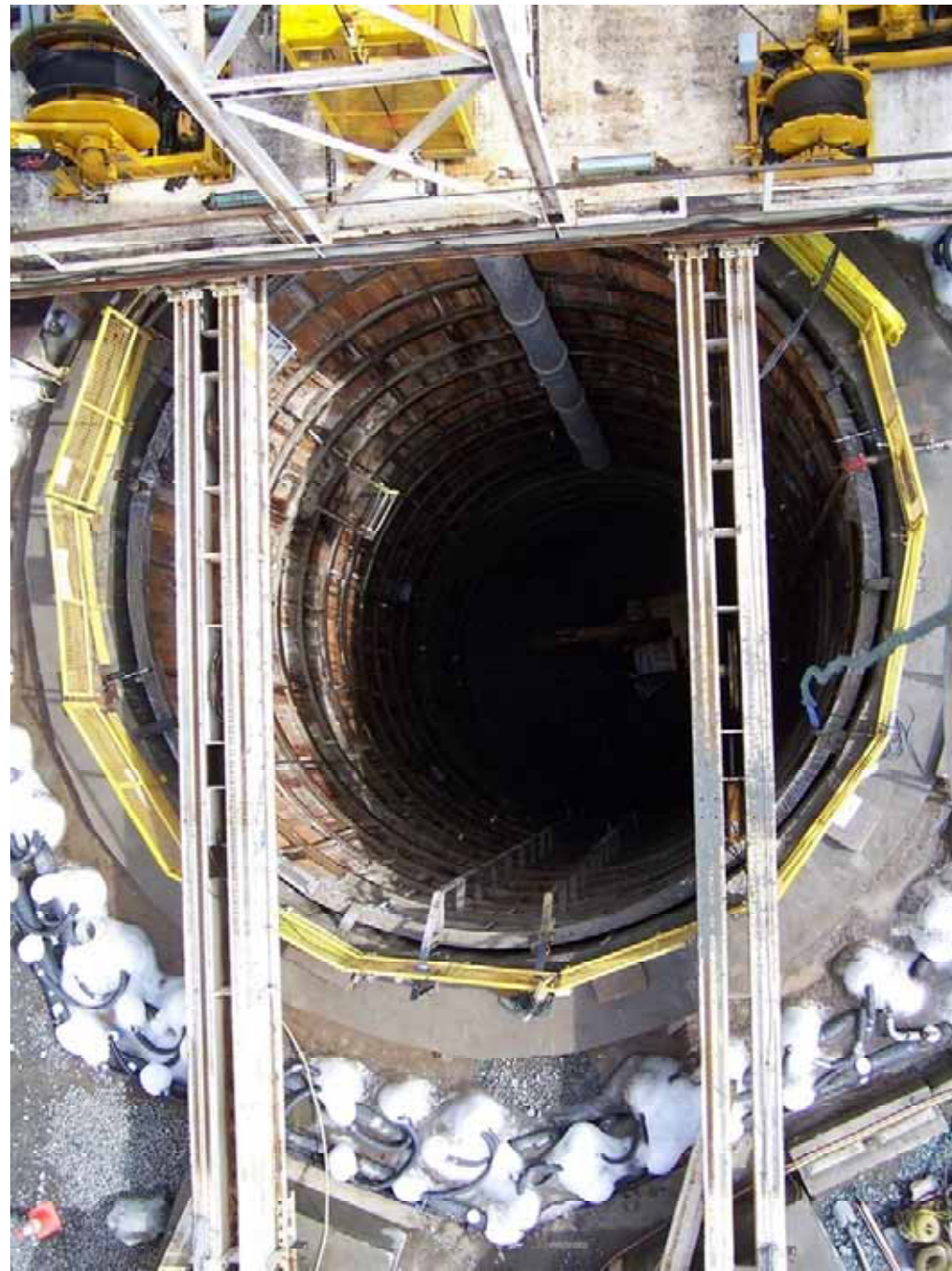
Figure 17. Freeze Shaft Excavation Near Completion
