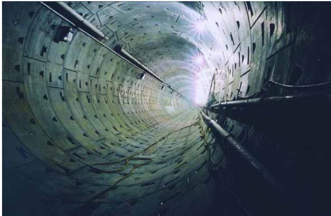
Figure 22. Bolted and Gasketed Precast Segmental Lining
