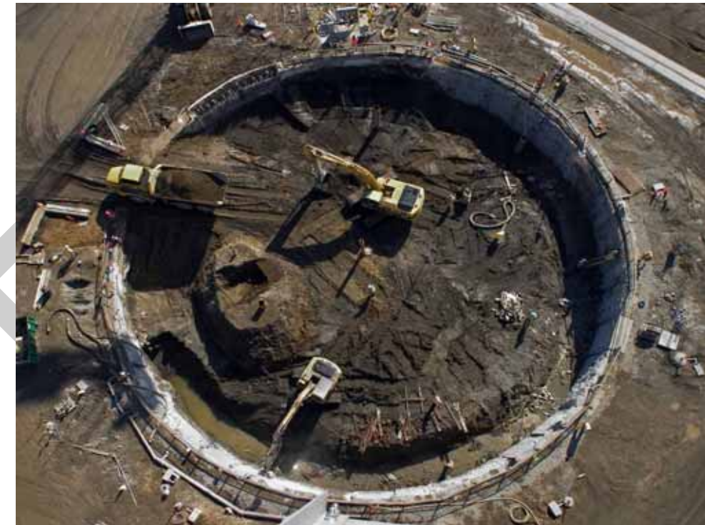
Figure 14. Slurry Wall Panels Complete and Ready for Interior Mass Excavation
