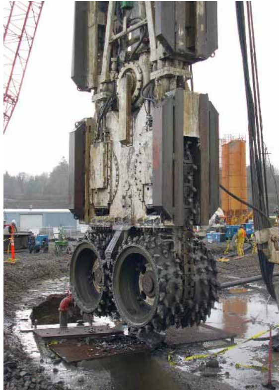
Figure 12. Hydromill used to Excavate Panels
