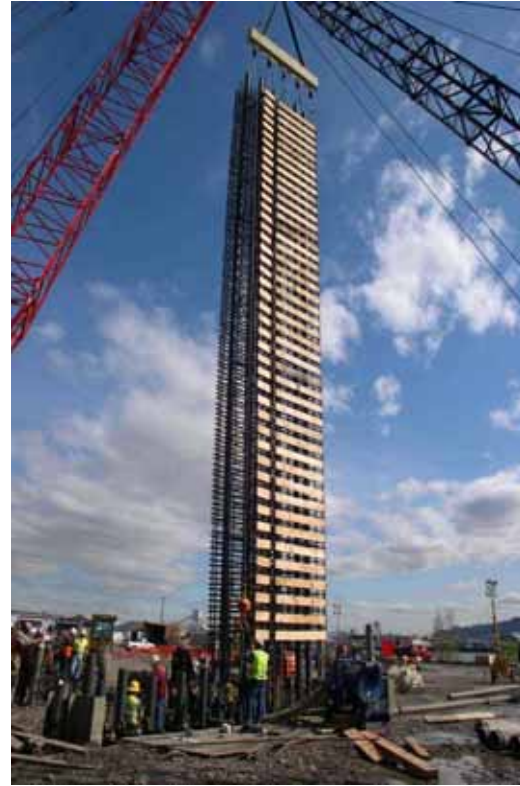
Figure 13. Slurry Wall Reinforcement
