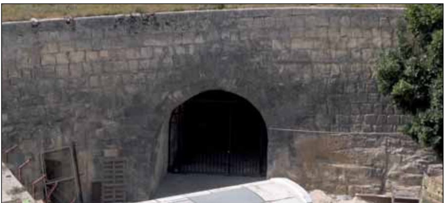
View of tunnel entrance in Fausse Braye
