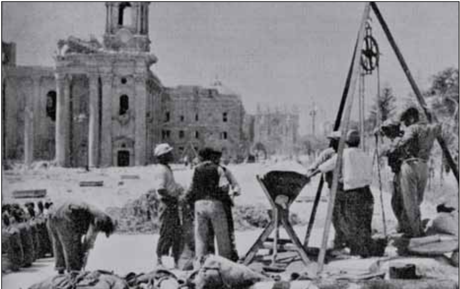
Damaged Parish Church and Granaries in use
