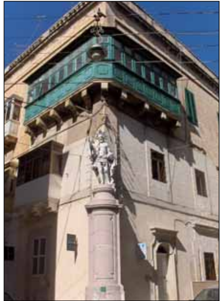
Corner Wooden Balcony
