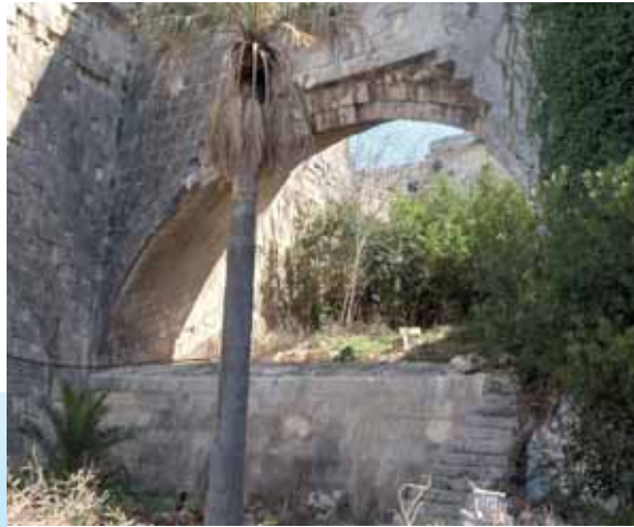
Skewed Arch at lower end of Sa Maison
