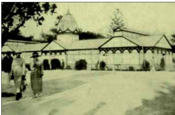
Former greenhouse in garden
