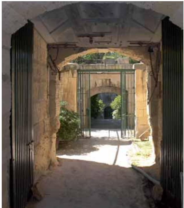
Raised iron door in ramp
