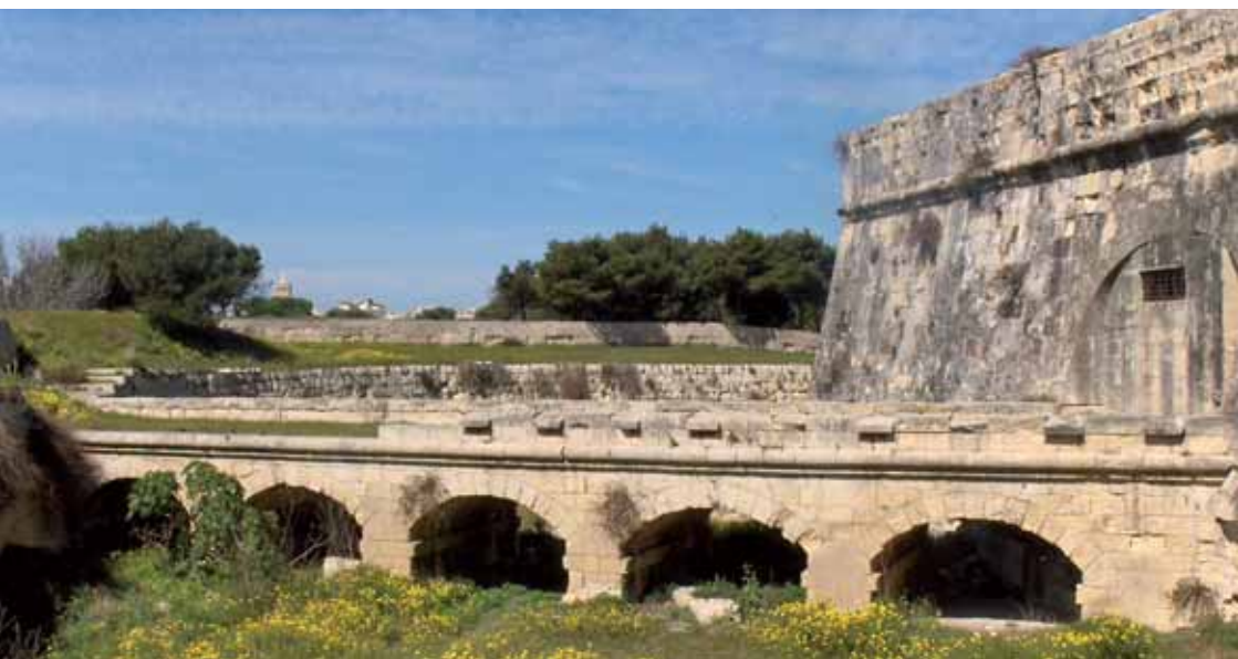
Tunnel exit on Viaduct
