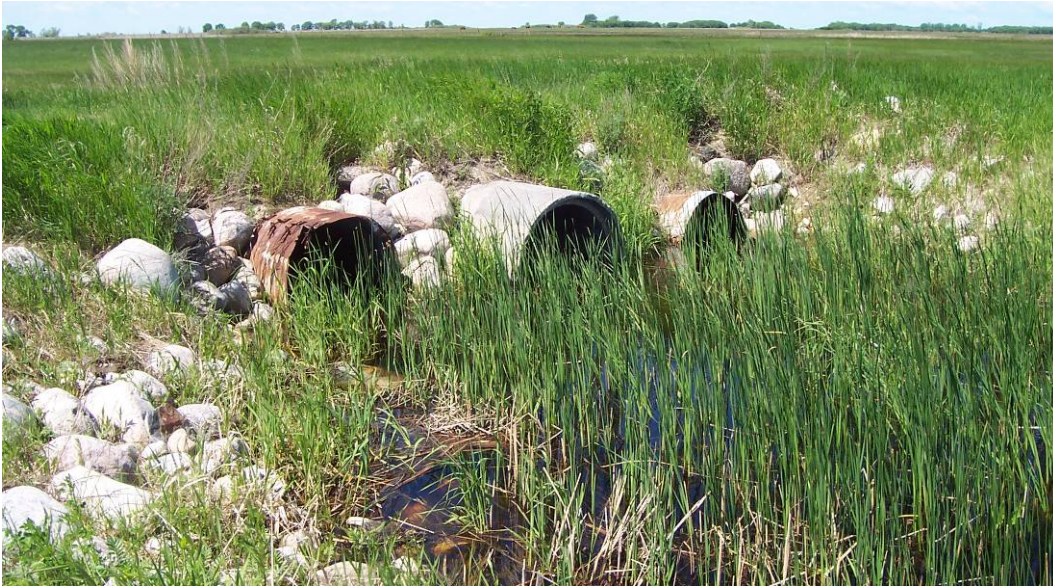
Photo 3.9 – Drain and Culvert near Lake Manitoba
