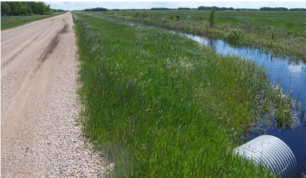
Photo 3.8 – Drain along South side of Wagon Creek Rd
