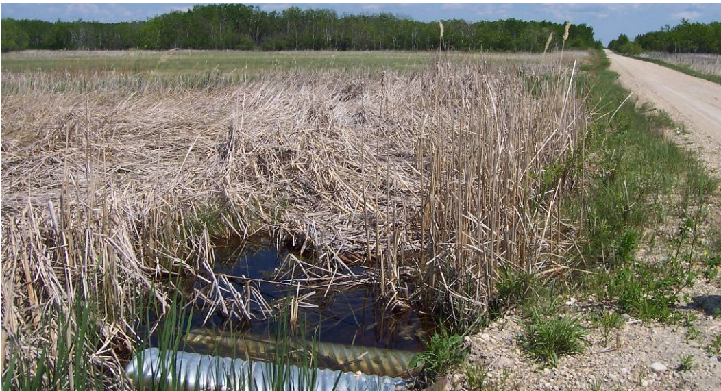
Photo 3.6 – Culvert crossing and Marshland along North side of Gaudry Rd
