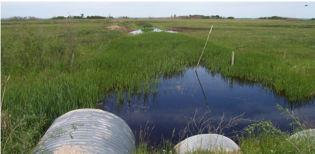
Photo 3.10 – Swamp Lake Drain (between PR 518 and West Shoal Lake)
