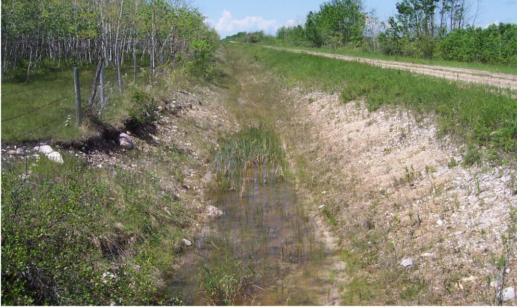
Photo 3.2 – Drain along South side of the Edmoudos/Boundary Rd near PTH 6
