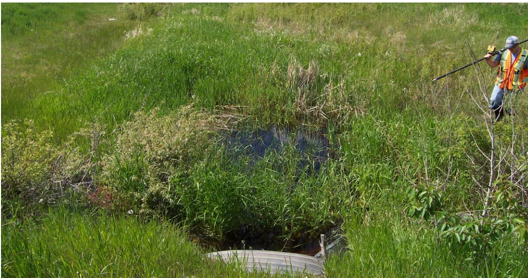
Photo 3.3 – Drain along East side of the PTH 6
