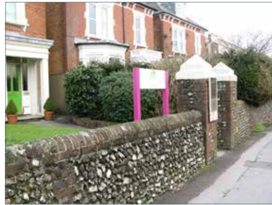
Flint wall in Station Road
