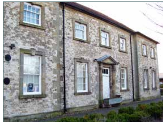
The former stables to Petersfield House, now a doctors' surgery
