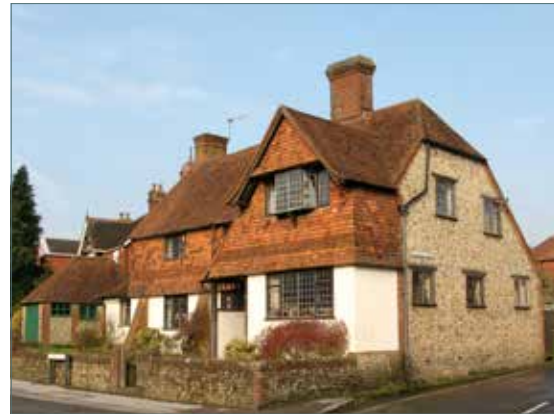
No. 16 Station Road
