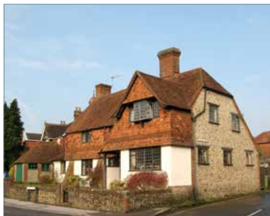
No. 16 Station Road
