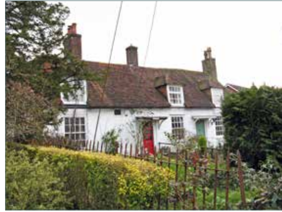
Nos. 63 and 65 Chapel Street
