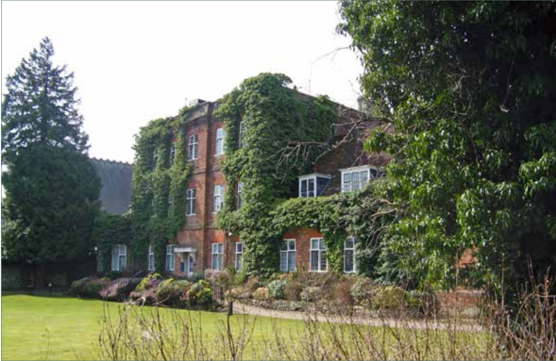
Rear view of The Old College, showing the different window pattern
