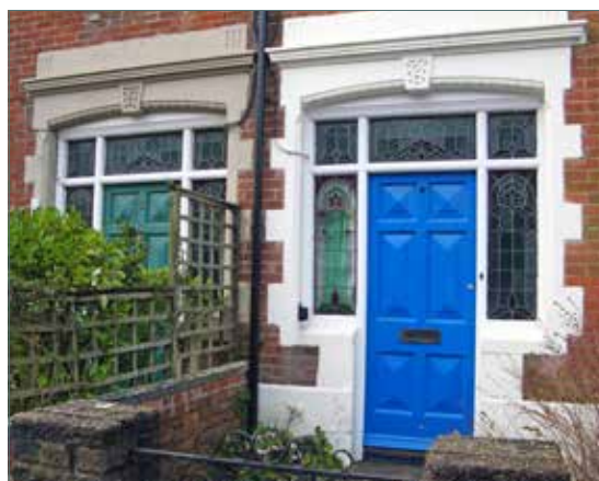
Sandringham Road front doors to Nos. 2 and 4
