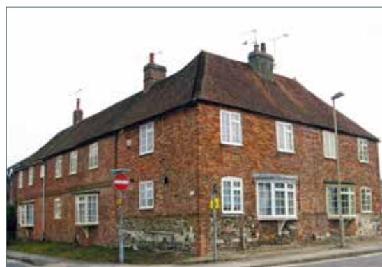
The Jolliffe almshouses in Swan Street
