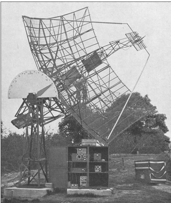
Figure 2: The 16 x 18-ft paraboloid at Georges Heights field station. It was proposed to ship this aerial to Brazil for the 1947 total solar eclipse (courtesy ATNF Historical Photographic Archive: B1164).
