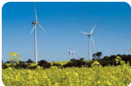
Springtime Canola fields and wind turbines, Collgar Wind Farm, Merredin
