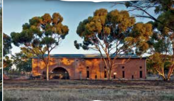
No 4 Pump Station, Merredin
