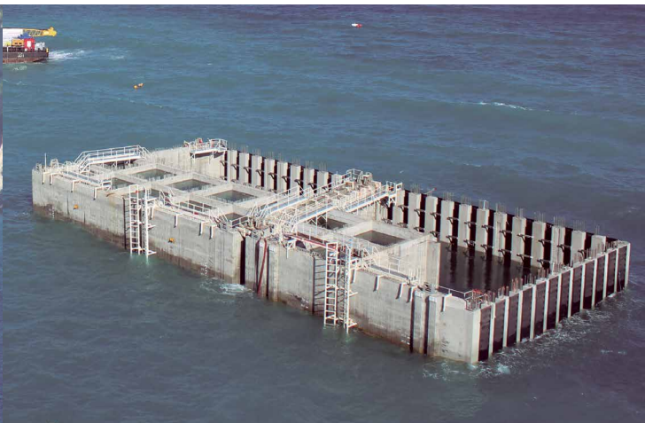
Caissons towed by boat to Monaco
