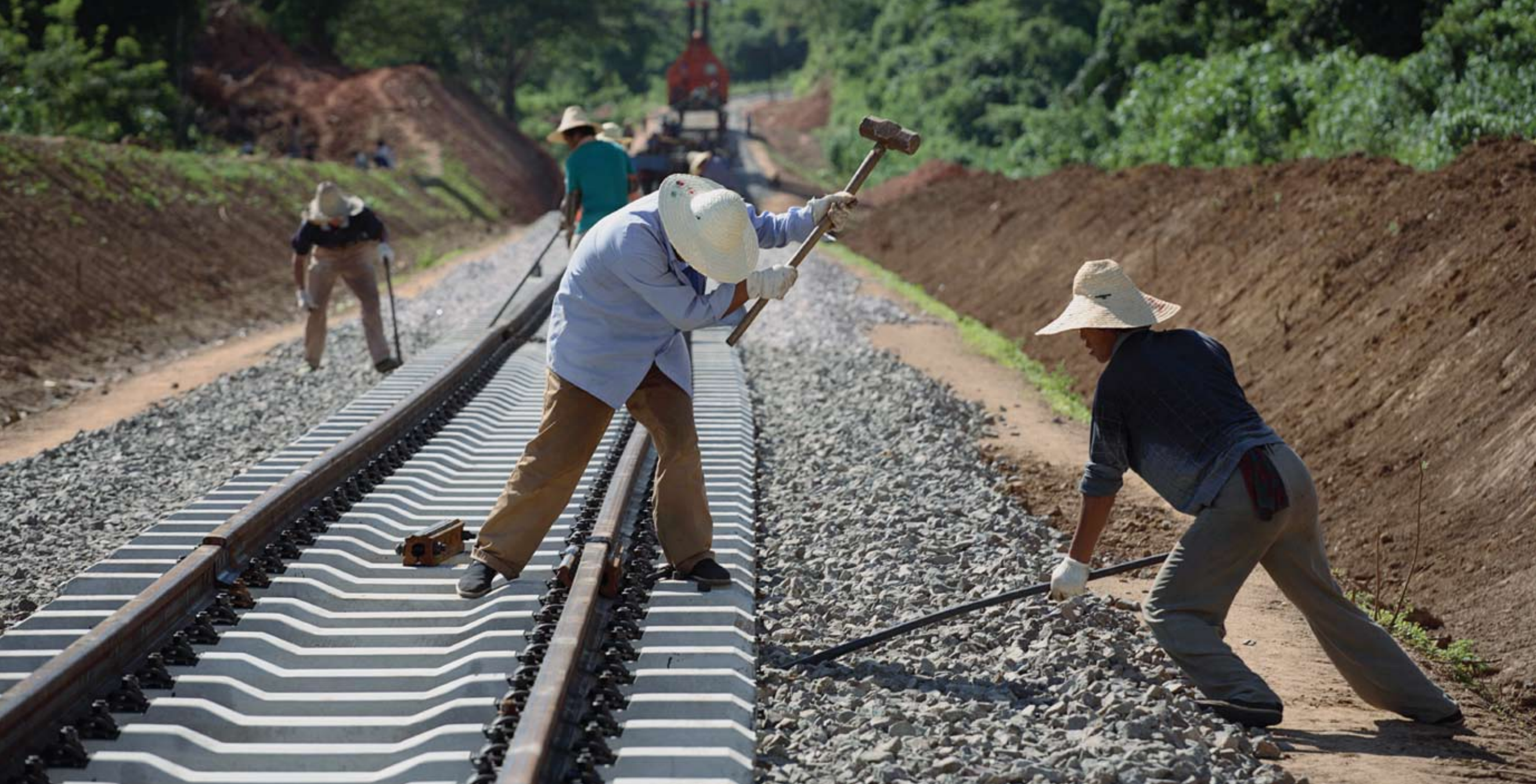
Chinese workers building railways
