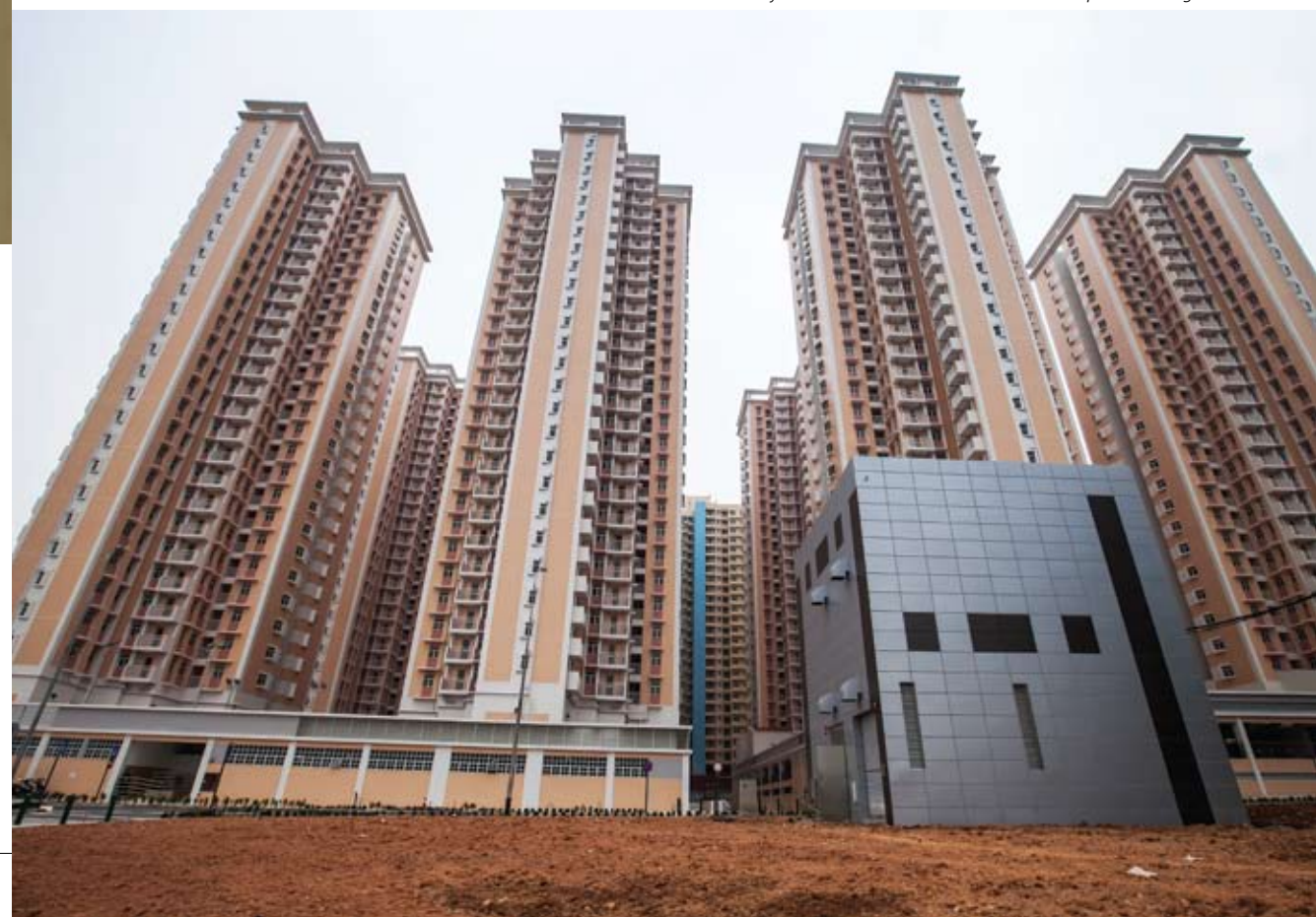
Recycled water installations in the Seac Pai Van public housing estate
