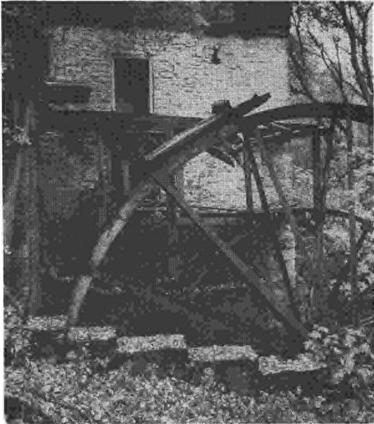
A corner of Thomas Shepherd's Grist Mill, off lower High Street, two stories of stone, 60 by 45 feet, showing water wheel 40 feet in diameter. Photo by Bodine.
