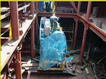
Hoisting the new main engines on board
