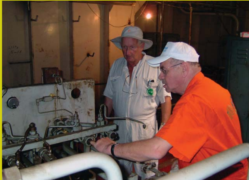
Inspection of part of the hydraulic installation
