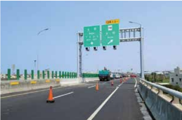
Daan Trunk Line Overpass Project in Fangli, West Coast Expressway (Provincial Highway No. 61)
