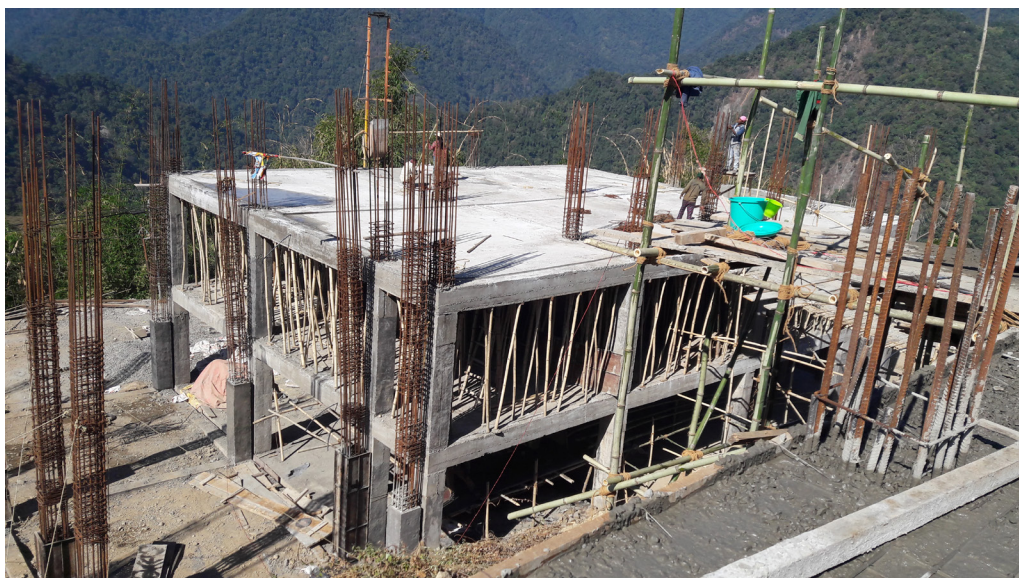
Electronics & Communication Laboratory Construction at Jigme Namgyel Engineering College
