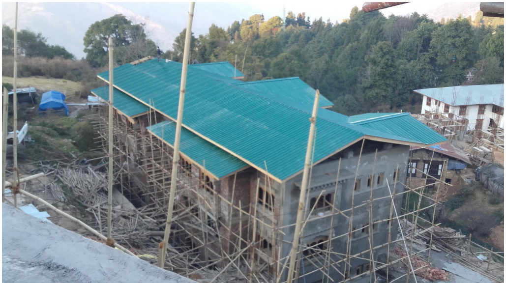
Student Hostel Construction at Sherubtse College
