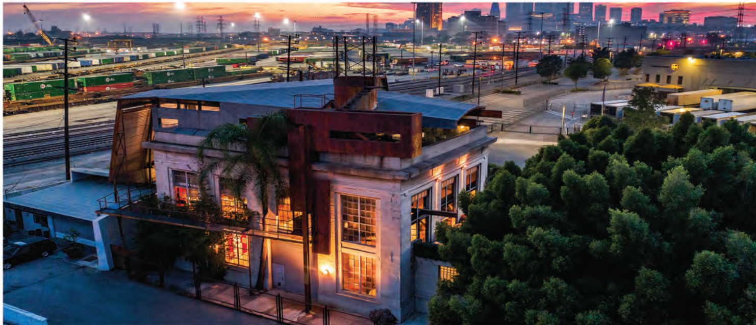
The Carlson-Reges Residence, 1922 698 Moulton Avenue, Los Angeles, CA 90031
