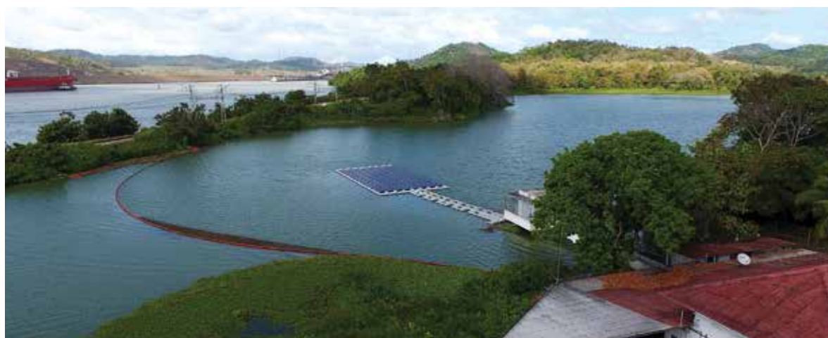
FIGURE 3.8. FPV system (with 24 kWp capacity) at Miraflores near the Panama Canal
