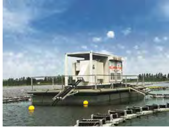
FIGURE 2.13. Sungrow FPV farm with a central inverter on a floating island (left), detailed view of the floating island for the central inverter (right)
