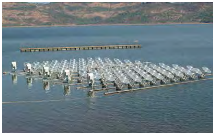
FIGURE 2.19. Sunengy's Liquid Solar Array with dual-axis tracking and concentrators (left), detail of the collector with lens concentrator (right), Whalvan Hydroelectric Dam, Lonavala, Maharashtra, India
