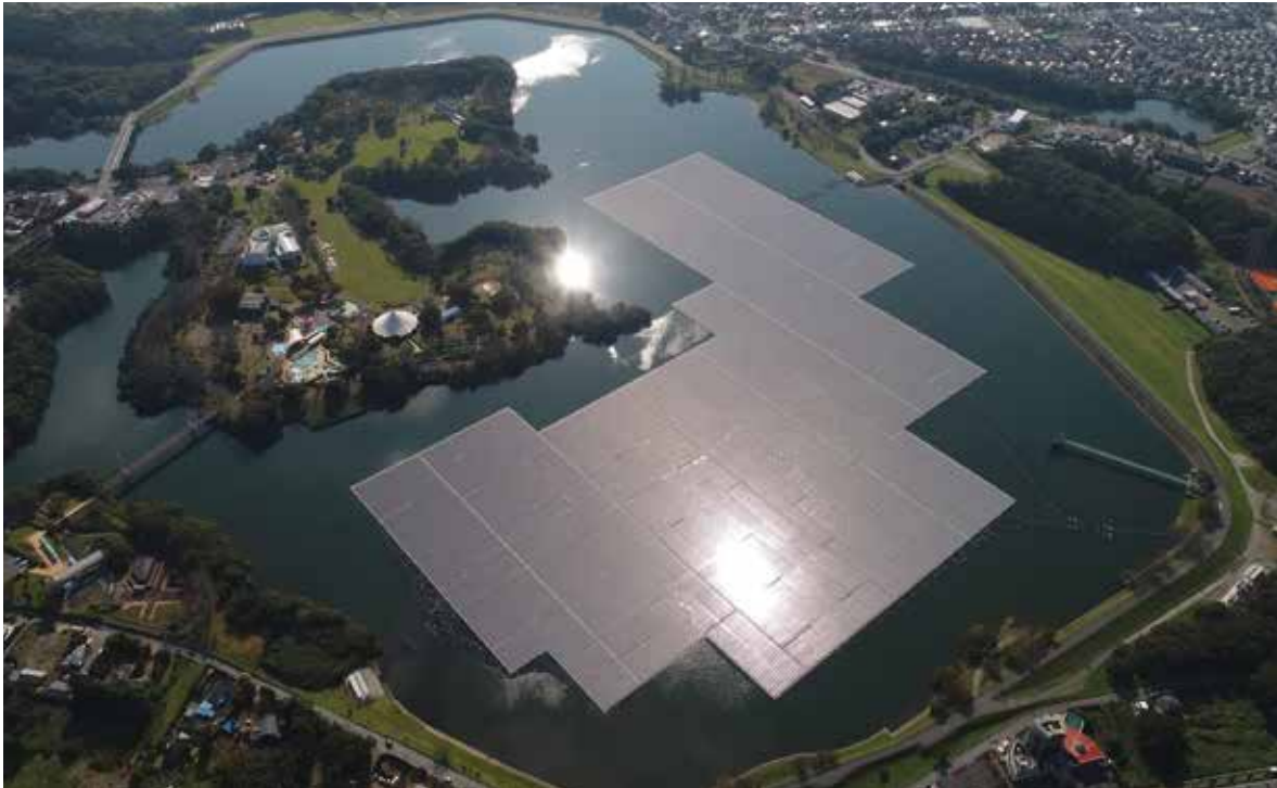
FIGURE 3.5. FPV installation (with a capacity of 13.7 MWp) at the Yamakura Dam in Japan
