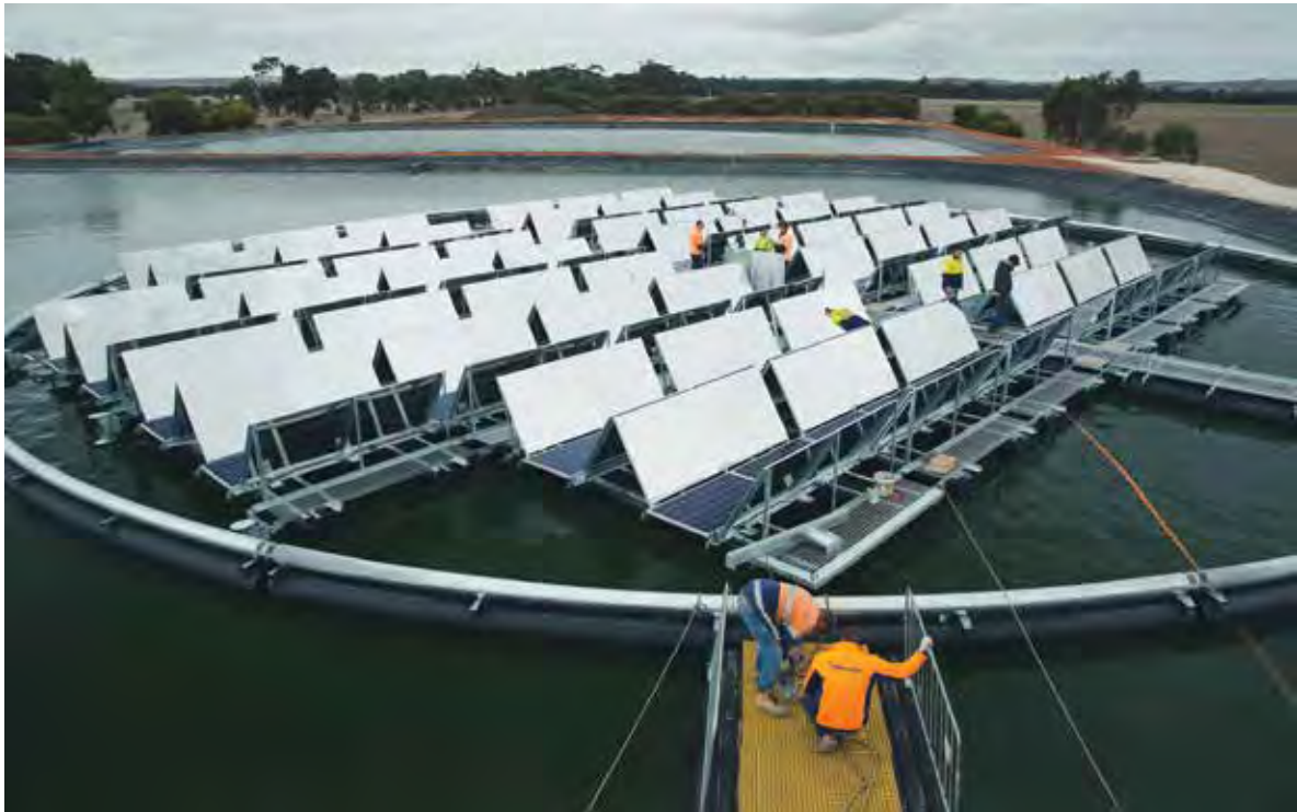
FIGURE 2.18. FPV with azimuth tracking (1-axis, vertical) in a wastewater facility, Jamestown, Australia
