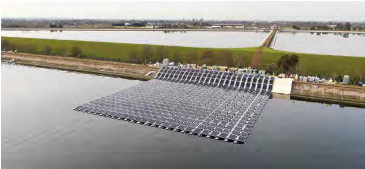
Source: © Lightsource BP Floating Solar Array, London.
