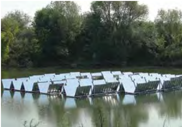
FIGURE 2.17. Low concentration with V-shaped mirrors for FPV
