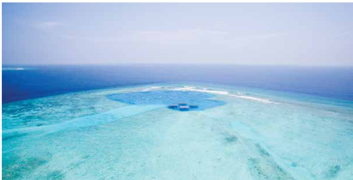
FIGURE 3.6. Offshore FPV system in the Maldives
