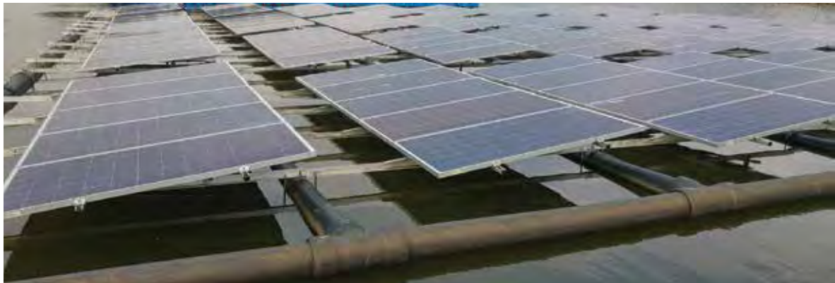
FIGURE 2.7. Various designs using metal frames and pipes to support PV panels, 4C Solar (top) and Koinè Multimedia (bottom)
