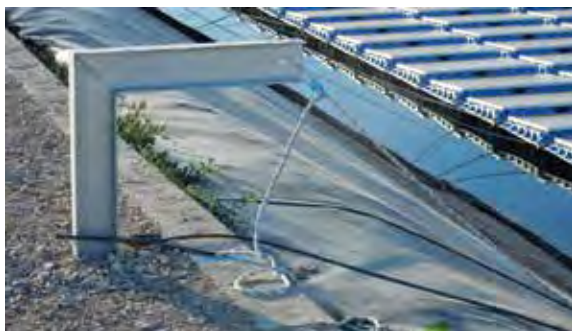
FIGURE 2.12. Bank anchoring example
