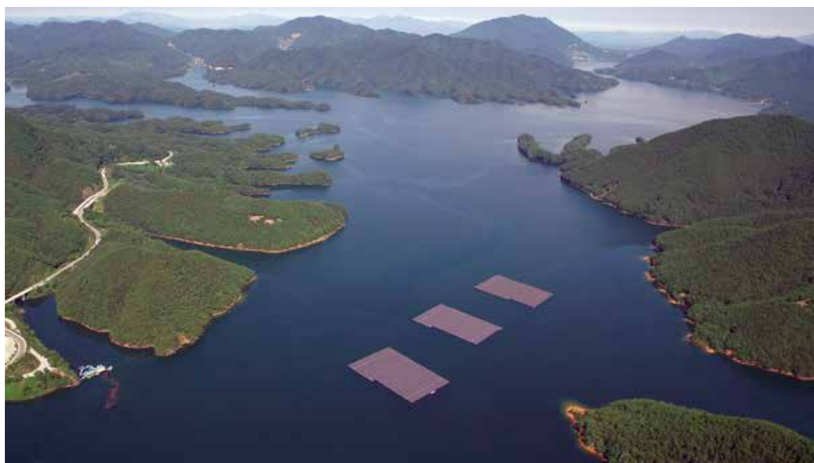
FIGURE 3.11. FPV installation (with a capacity of 3 MWp) Cheongpung Lake, Chungju Dam in Korea
