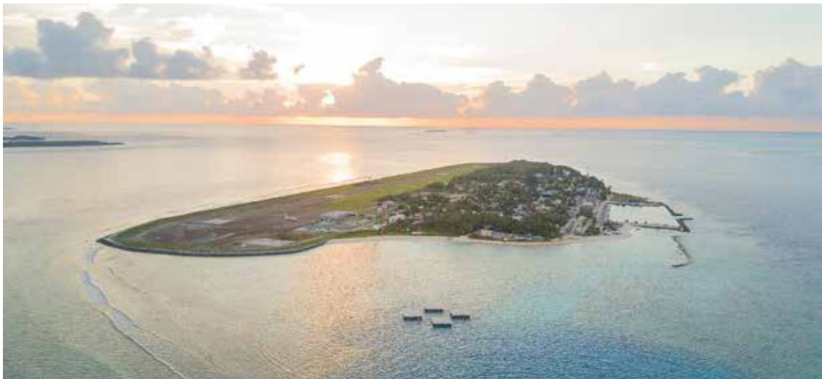
FIGURE 2.23. Swimsol's pilot offshore FPV plant on a resort island in the Maldives
