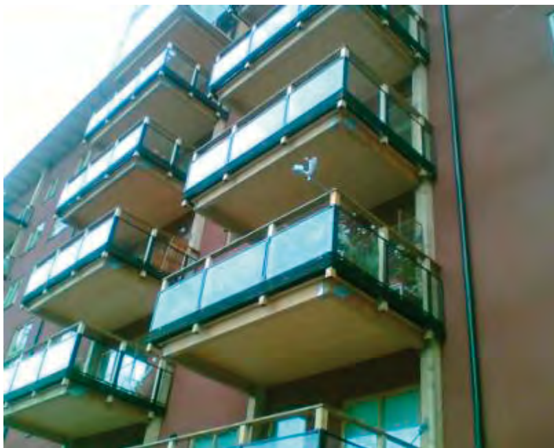
Figure 108: Prefixed balcony construction, source: Stora Enso company
