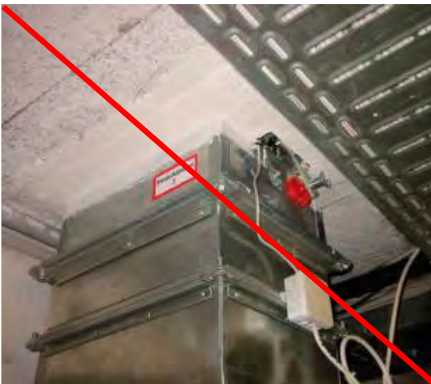
Figure 93: Installation of a fire protection flap in a soft partition without expansion compensation or rigid connection, source: Air Fire Tech company
