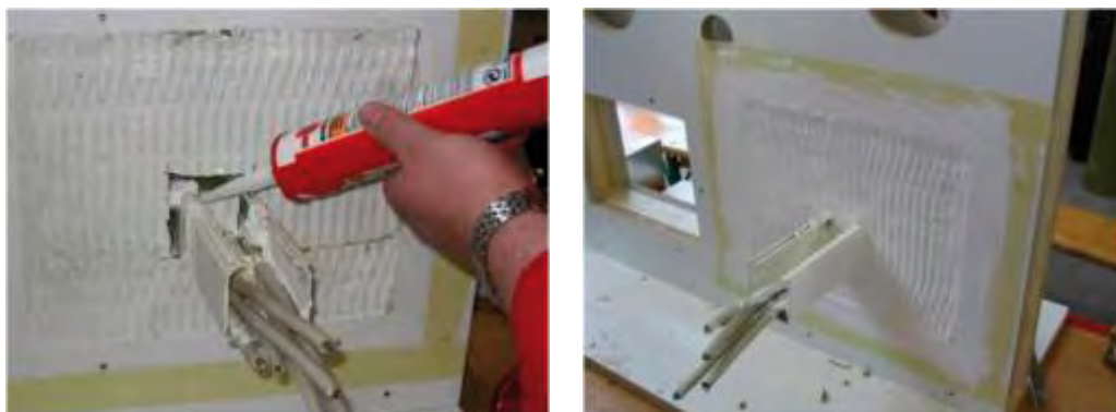
Figure 83: Sealing of cable penetrations and finished partitioning, source: Würth company
