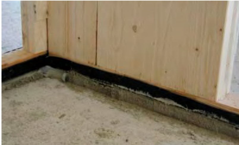
Figure 47: Support detail of an internal wall
