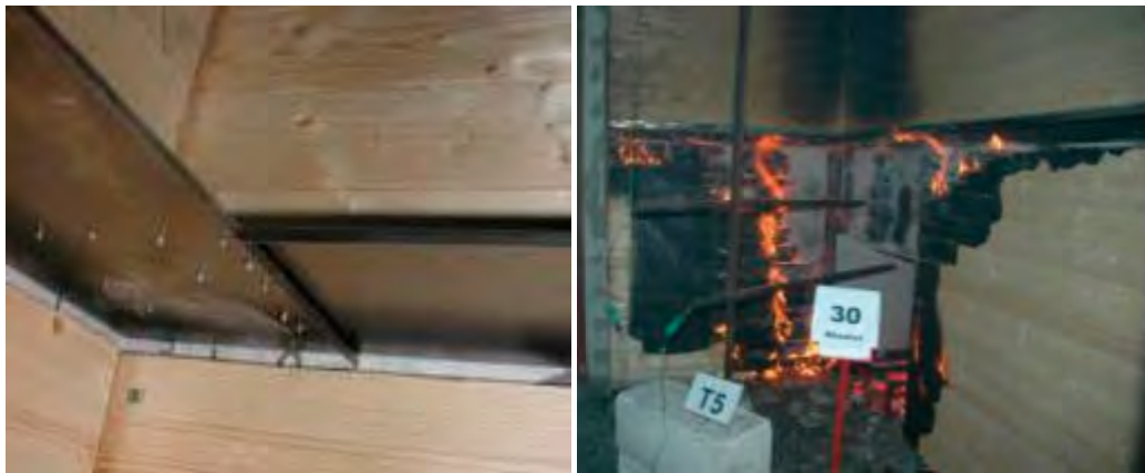
Figure 101: Implementation of an internal corner of a fire barrier and fire experiment at a façade with fire barrier
