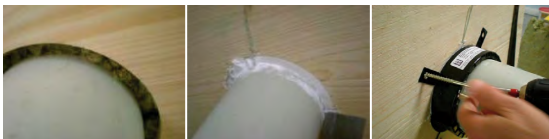
Figure 85: Installation of a fire protection collar directly in an unclad solid timber wall; left: Filling up the annular gap, center: intumescent fire protection compound, right: fastening of the fire protection collar
