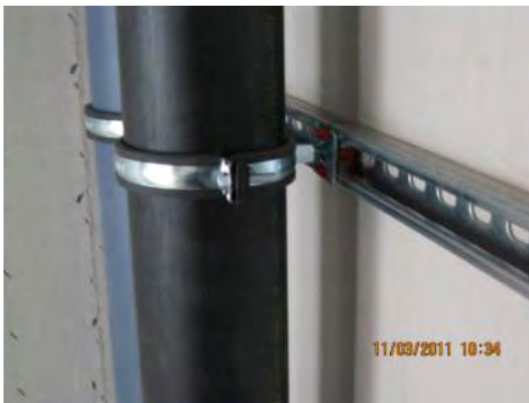
Figure 78: Sound protection decoupling of pipes
