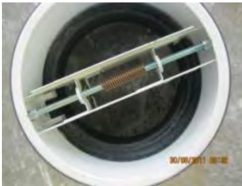
Figure 87: View of a fire protection closure based on intumescent materials with closing element (FLI-VE)
