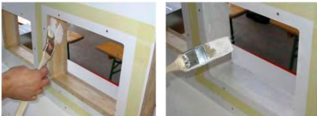
Figure 81: Application of coating on reveal and reveal coating, source: Würth company
