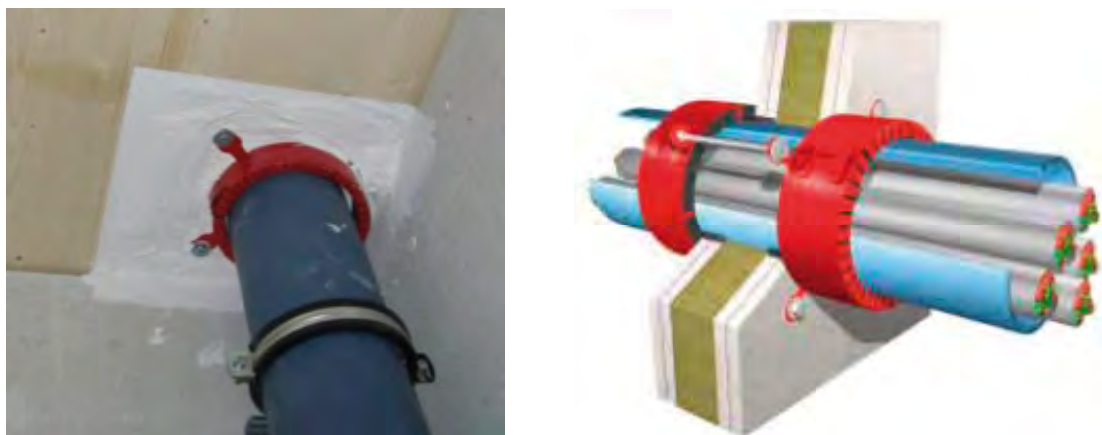
Figure 86: Fastening of a fire protection collar in a soft partition is admissible only if it is led through, source: bip company
