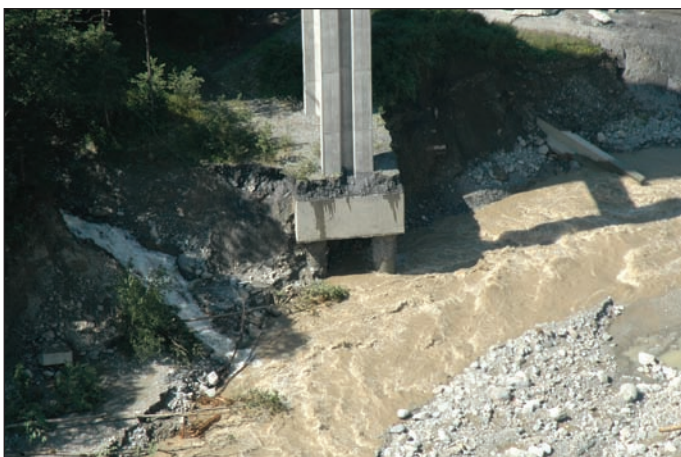
Fig. 3: Uncovered pile cap of pier P3
