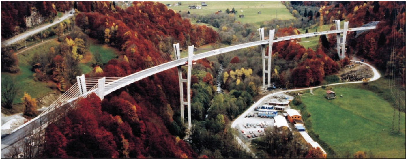
Fig. 1: Sunniberg Bridge after completion in fall 1998 3
