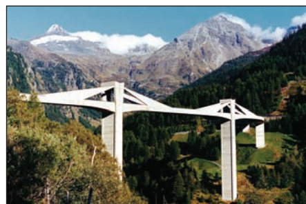
Fig. 5: Ganter Bridge by Christian Menn
