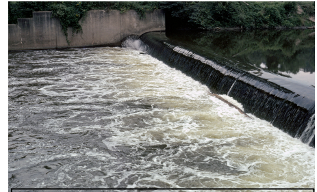
Brecksville Dam, built 1952
