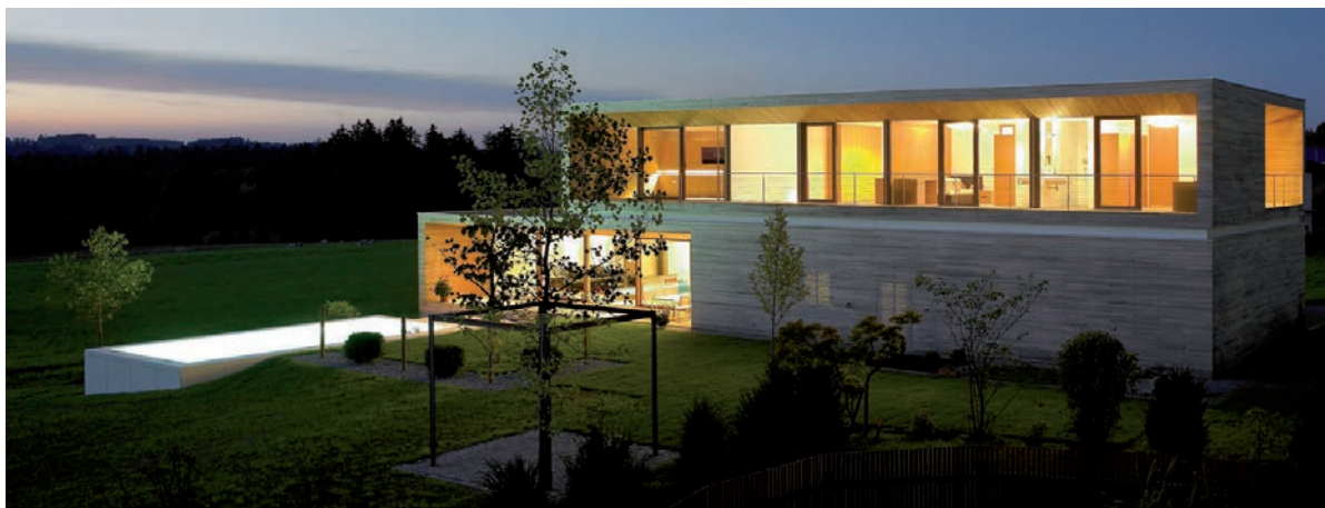
Vorarlberg wood construction creates aesthetic accents throughout the local landscape. This image features a single-family home in Hörbranz, designed by Jürgen Hagspiel. ©Hagspiel, VlbG. Wood Construction Award | TOP The System3 modular home impressed visitors to New York's MOMA. ©B.Tse
