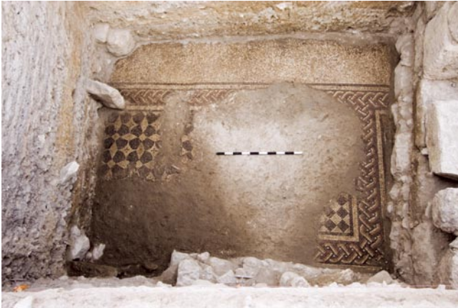
Late Roman mosaic floor as disturbed by Byzantine structures in Area XXXIIIBB looking from above
