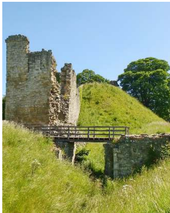
Fig. 78. Pickering Castle. A royal castle. It received its stone shell keep c. 1220. The screen wall protects the stair approach to the keep. Image: Neil Guy.
