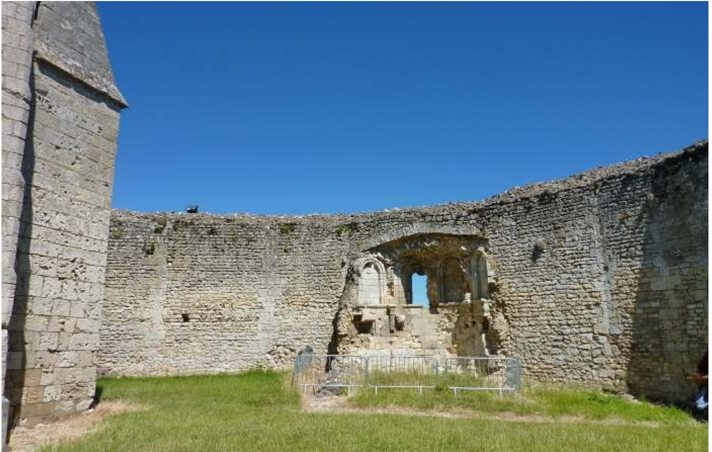
ABOVE: Fig. 59. Gisors Castle. Looking east. Central shell, with polygonal inner tower left, and chapel apse directly ahead.
