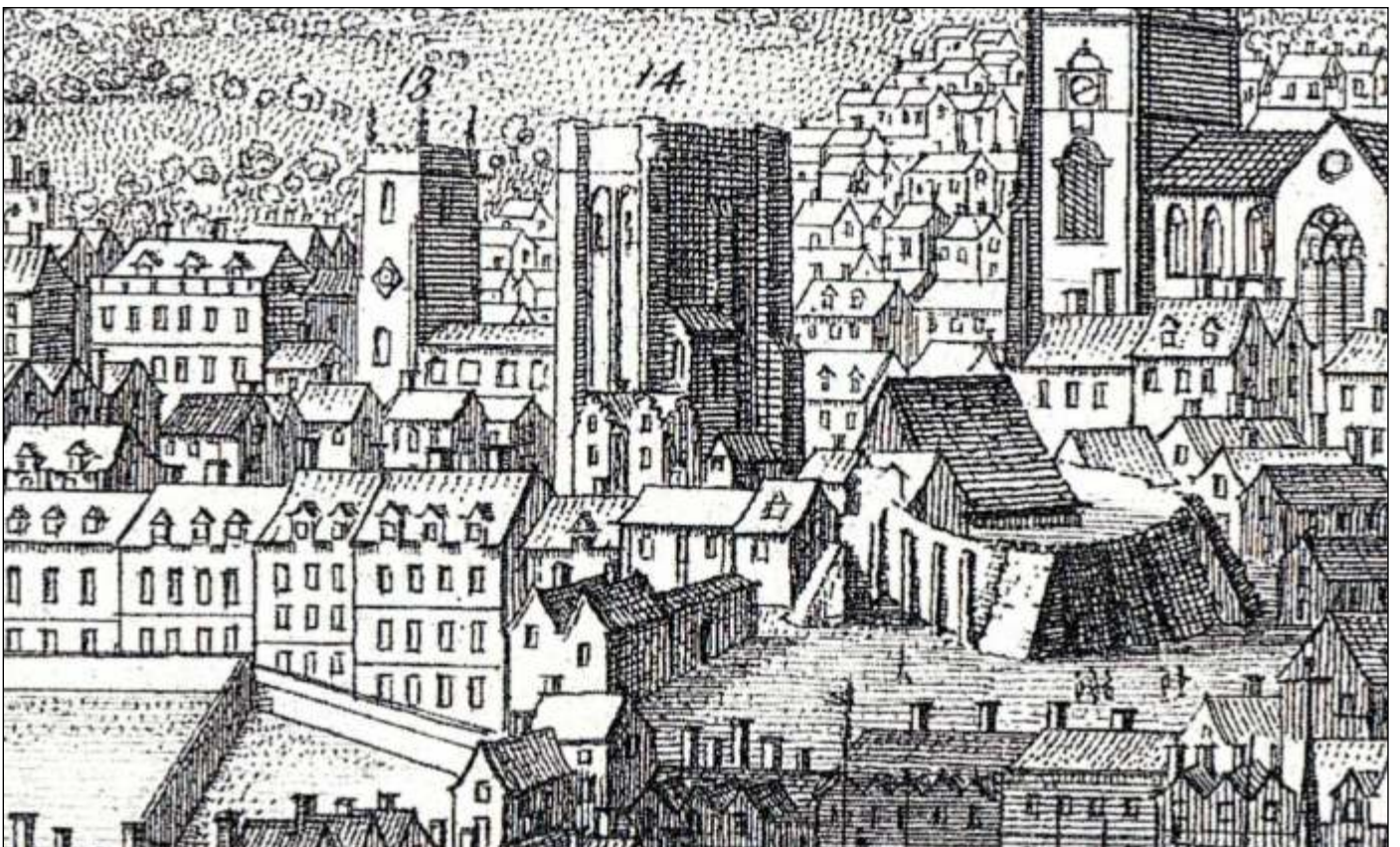
BELOW: Fig. 20. 'The South-East Prospect of Newcastle upon Tyne'. From Samuel and Nathaniel Buck's Town Prospects , c. 1723, showing the Great Tower, the revetted and buttressed 'shell-keep' (or half-moon battery) to the east.
