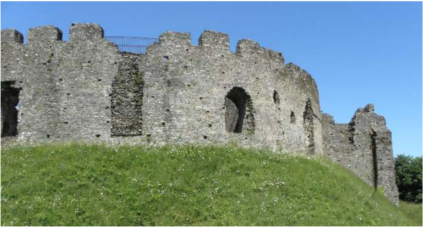
Fig. 74. Restormel Castle from the south, illustrating original exterior low-level hall windows, although within the courtyard the hall is at first-floor level. Image: Neil Guy.
