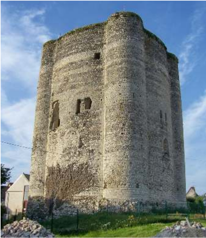
Fig. 66. Houdan Castle c. 1130. Square interior with splayed corners but on the outside circular with four projecting turrets. Source: Henry Salomé, via wikipedia Creative Commons Attribution-Share Alike 3.0 Unported
