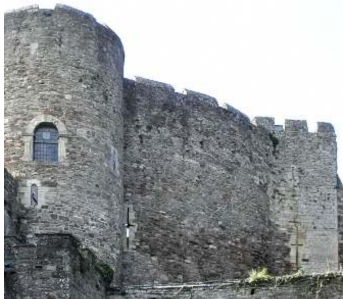
Fig. 50. Berkeley Castle. Shell-keep, N-E side, over 40ft high. Three cruciform 'arrow slits' visible on or adjacent to the lobed towers. See (o) 'Defensive features'. Image: Neil Guy.
