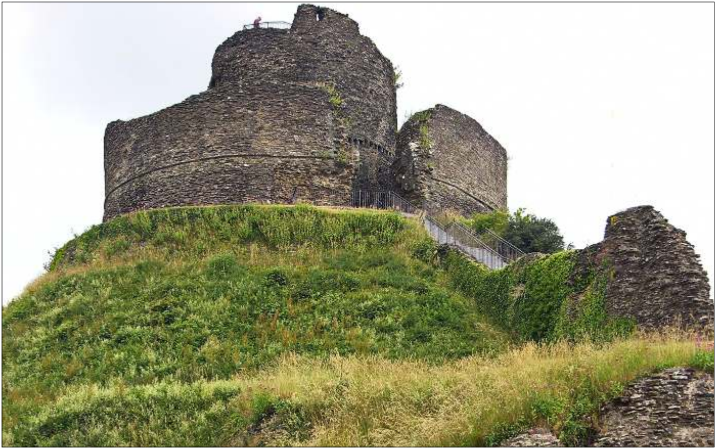
ABOVE: Fig. 33. Launceston Castle, showing the later circular donjon within the earlier outer shell-wall. Image © Author.
