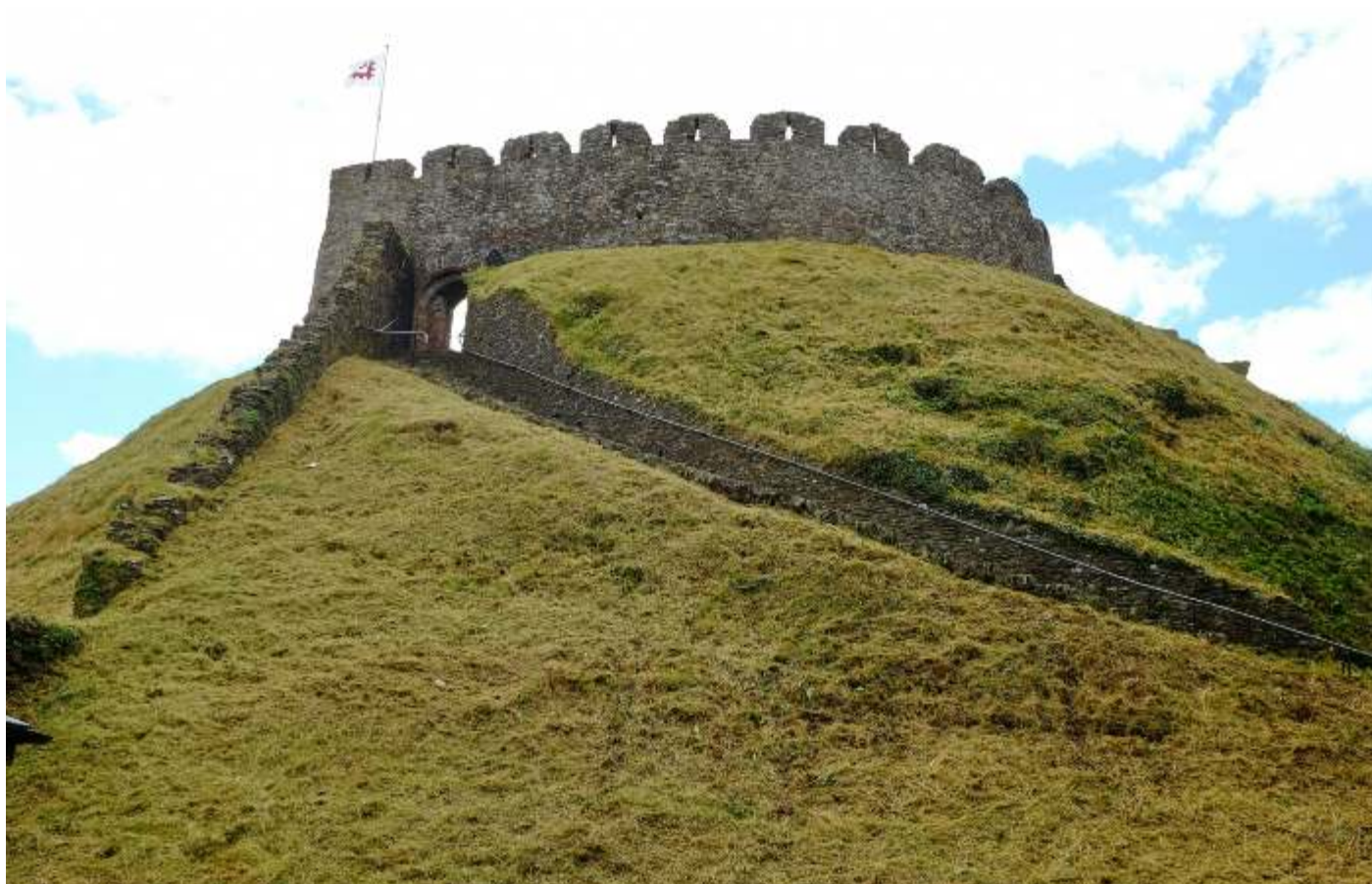
Fig. 52. Totnes Castle. The shell-keep from the inner bailey, (from the north). The present diagonal path up to the entrance post-dates the infilling of the ditch. The entrance is sheltered by the eastern wing wall (left). (See page 39). Details of the internal layout are also discussed and illustrated in the Catalogue entry for Totnes. Image: From the Author's collection.
