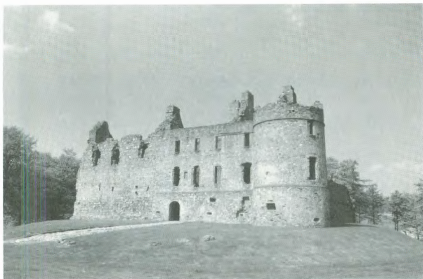
Fig.11.4 Balvenie Castle, Dufftown. Mid sixteenth century facade. (E Beaton)
