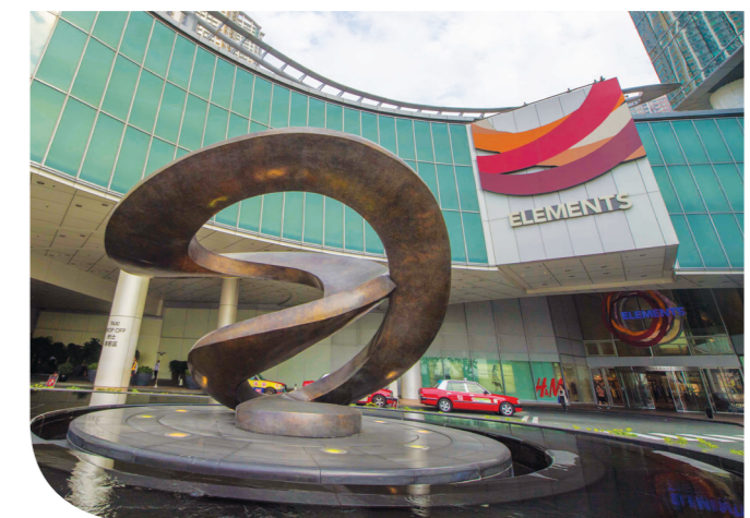
The Corporation's flagship shopping mall, ELEMENTS, atop Kowloon Station.
