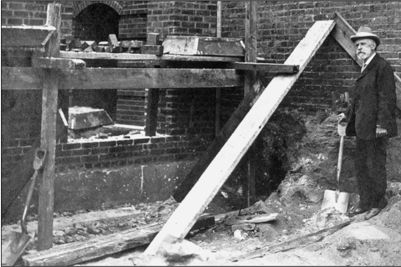
Frederick Putnam breaking ground for the 1913 addition.
