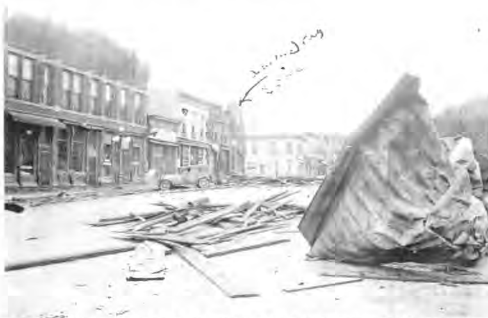
Figure 1 Storm damage, 1934. The crumpled heap of material in the right foreground is the pressed metal cornice from the Union Drug building noted in the background. From a newspaper clipping in the collection of Richard O. Woodard.
