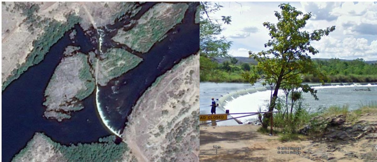
Figure 12. Ivanhoe Crossing, a concrete causeway across the main channel of the lower Ord River, Western Australia.
