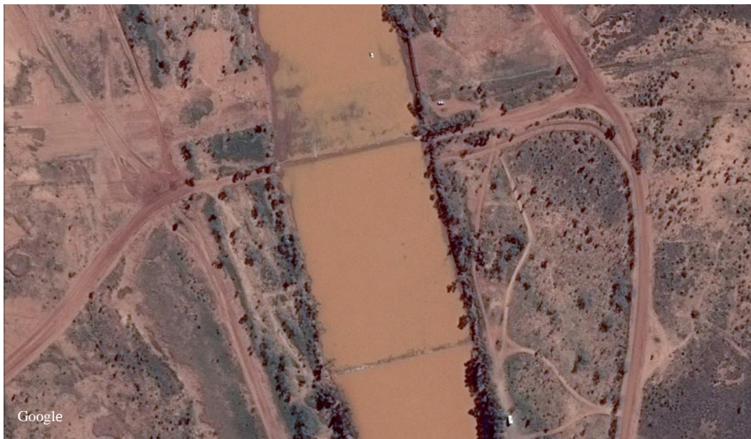
Figure 7. Two barriers across the lower Ashburton River
