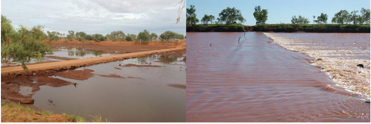
Figure 16. The Ashburton Crossing (a) after high tide and (b) during a high flow even in April 2011.
