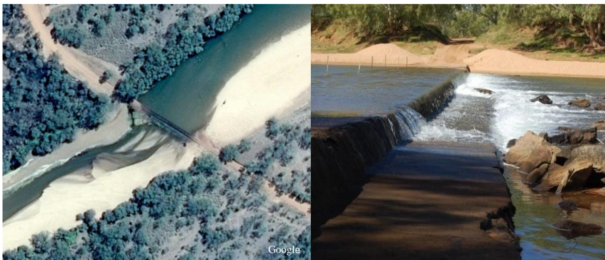
Figure 10. Myroodah Crossing, a concrete causeway across the main channel of the Fitzroy River, Western Australia.
