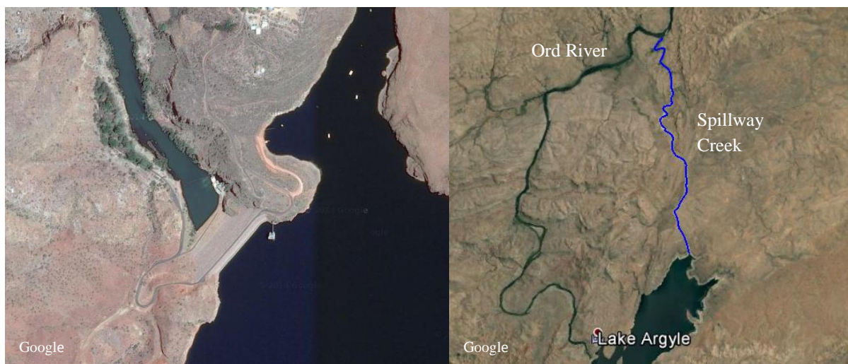
Figure 14. (left) Lake Argyle Dam on the main channel and (right) the potential bypass (Spillway Creek) of the Lake Argyle Dam on the Ord River, Western Australia.
