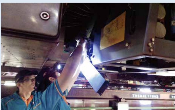
空壓機模組檢修 Overhaul on air compressor module
