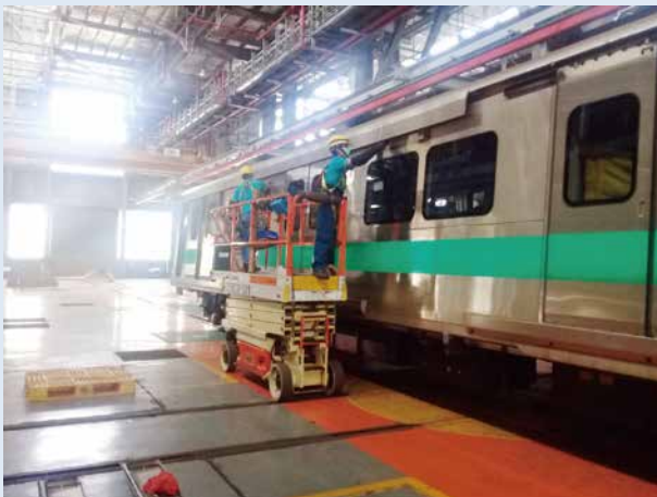
排水槽車門導軌潤滑 Lubricate drainage channel and door rail
