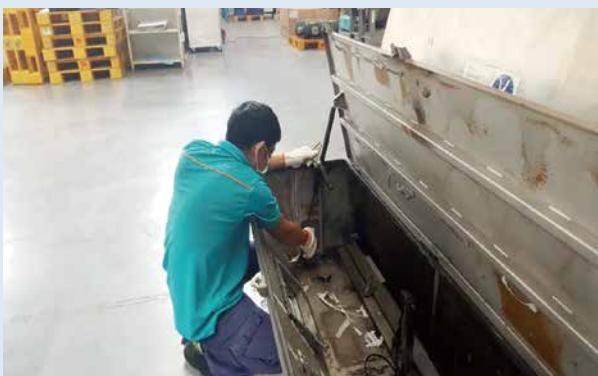
空調機組隔熱棉更換 Replace air-conditioning unit insulation cotton
