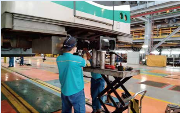
自動聯結器檢修 Overhaul on automatic connector
