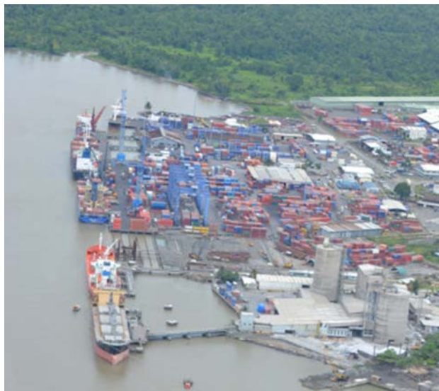
Lae Container and Bulk Vessels Berths
