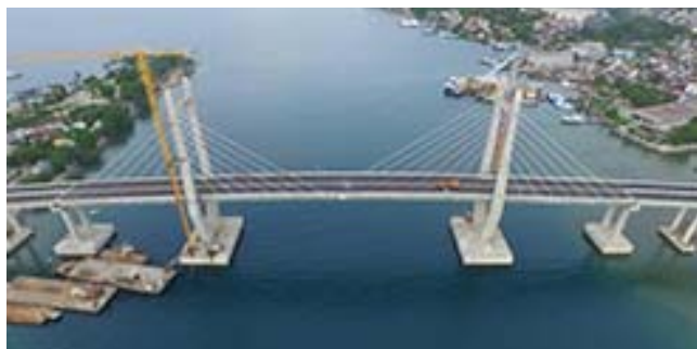
Merah Putih Bridge in Ambon Bay entrance
