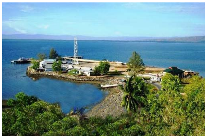
Namlea Light and Port in Pulau Buru
