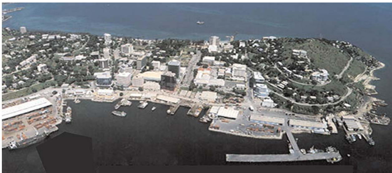
Port Moresby—Main Wharf facing SE
