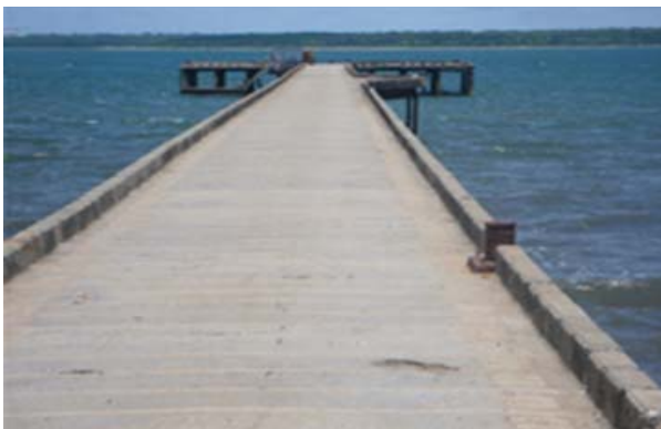
Port of Daru Pier
