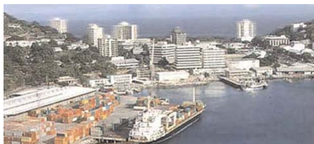
Port Moresby Container Terminal
