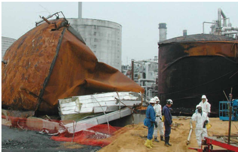
Aboveground storage tank explosion, Delaware, 2001.
