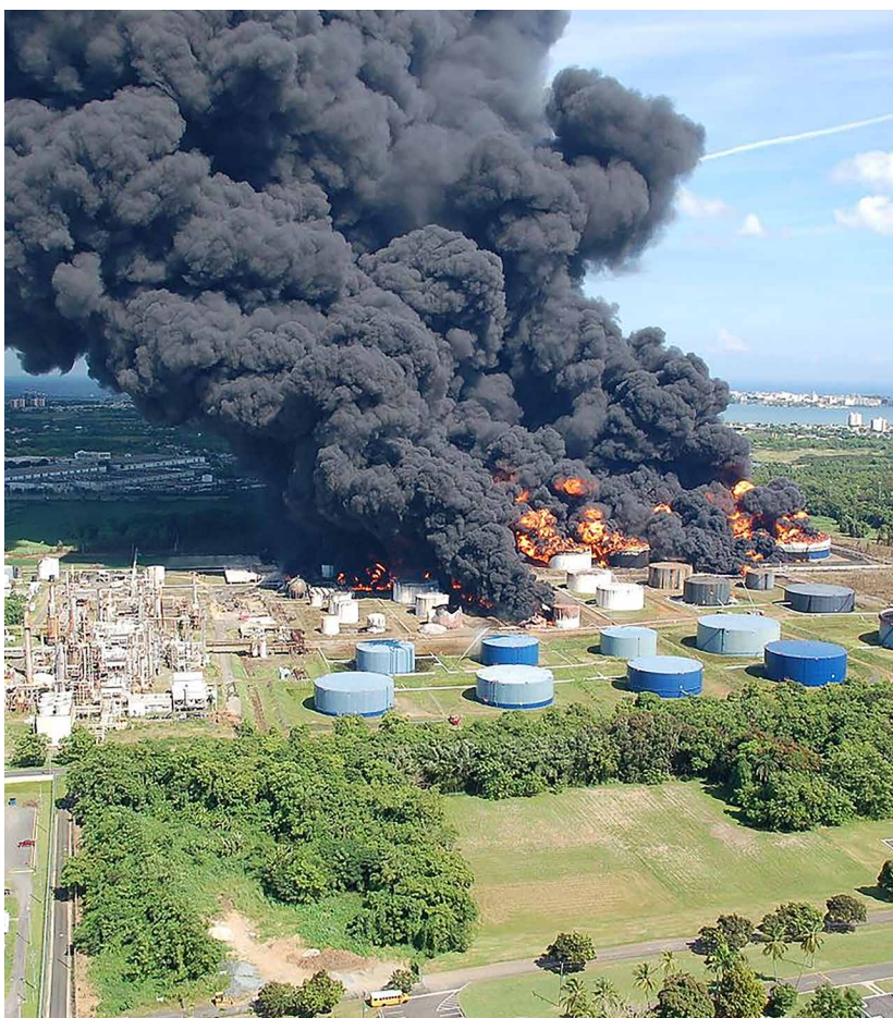
Caribbean Petroleum Corporation storage tank explosion and fire in Puerto Rico. 34
