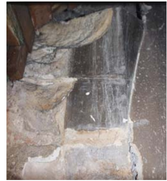
View of the arch-spring over the corbel above Test Pit 5
