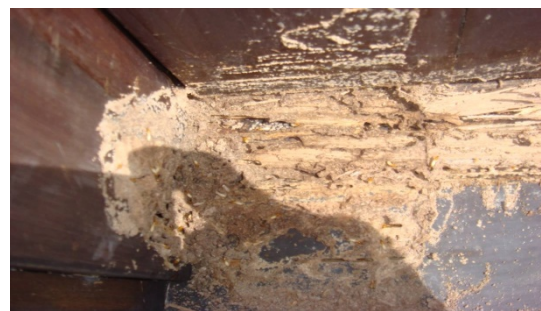
Figure 4. Sign of Coptoteremes damaging kitchen door of villa 2090
