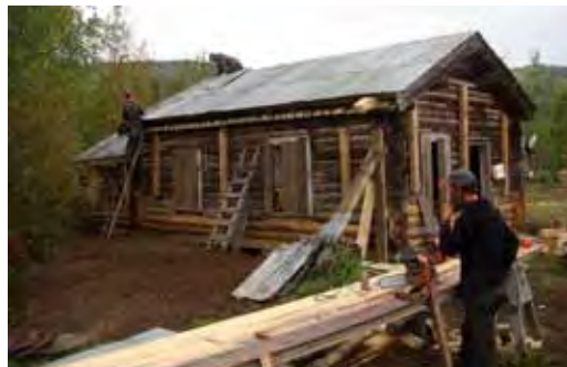
Stabilization and restoration work.
