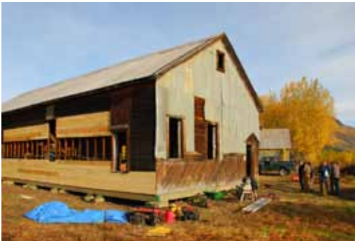
A restoration crew at the site in 2007.
