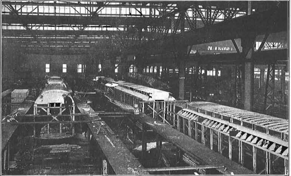
Portion of Passenger Car Erecting Department, Showing Interurban Cars in Course of Construction.
