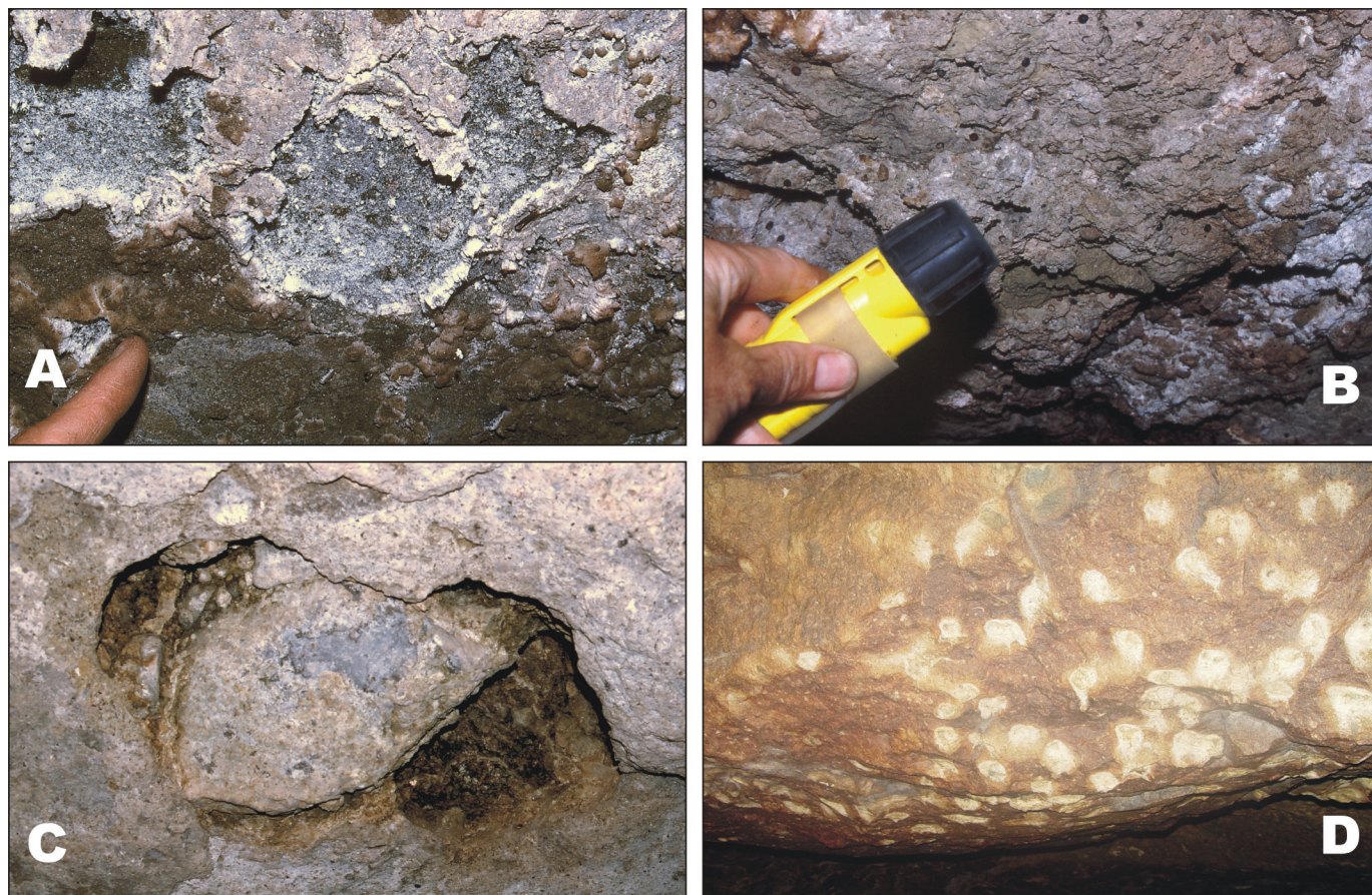
Figure 6. (A) Kitum Cave antechamber, close to entrance: Efflorescence flaking of ceiling and wall surfaces in grey agglomerate is shown. (B) Kitum Cave antechamber, close to back of the cave: Spongy carious weathering of ceiling in yellow-grey agglomerate. The rock is soft to a depth of at least 10 cm. (C) Mackingeny Cave: Weathered aureole around large clast in grey agglomerate (~50 cm wide); eventually the clast will fall leaving circular cavity in roof. (D) Mackingeny Cave: roof discoloration from bat roosting; white blobs are ~20 cm wide.
