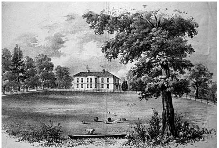
Kemnal House in its new position
