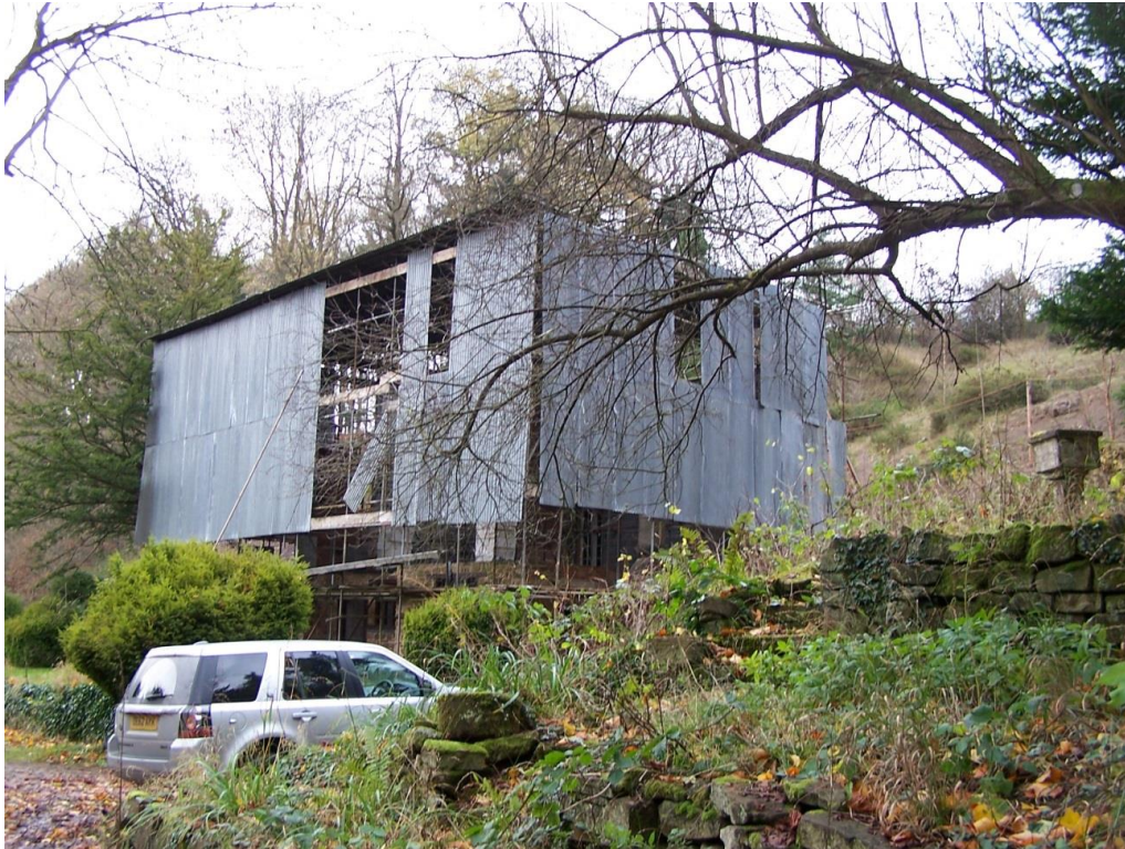
Dowles Manor House under protective sheeting
