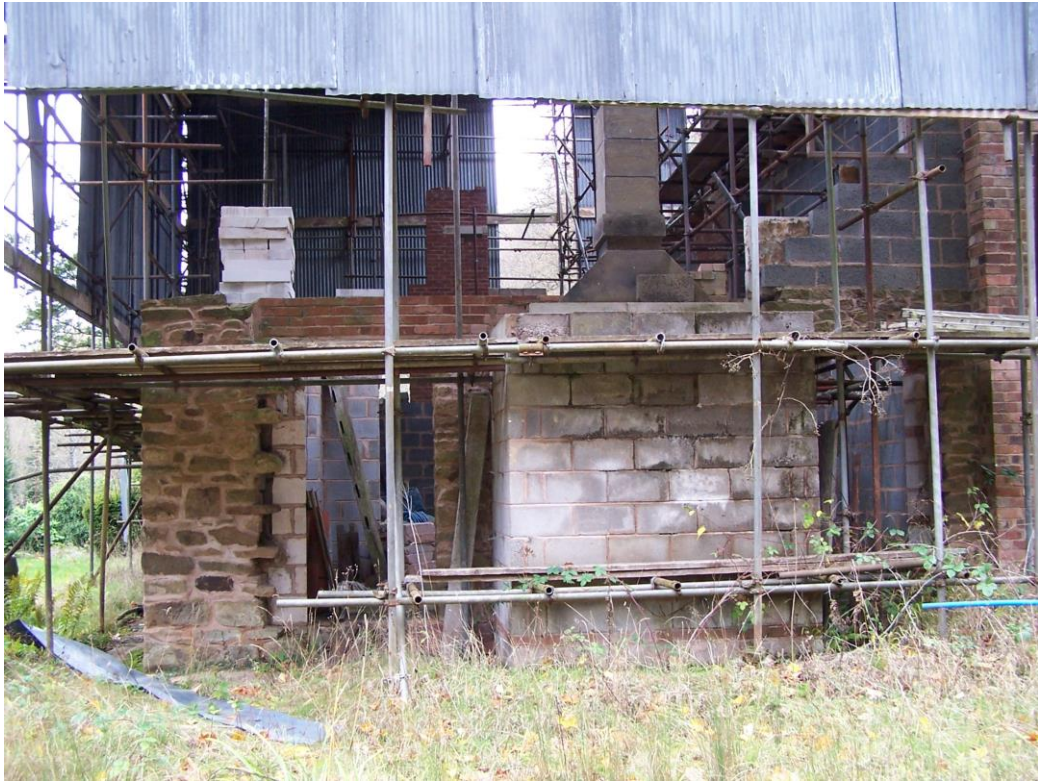
The front element of the Manor House is only partially rebuilt
