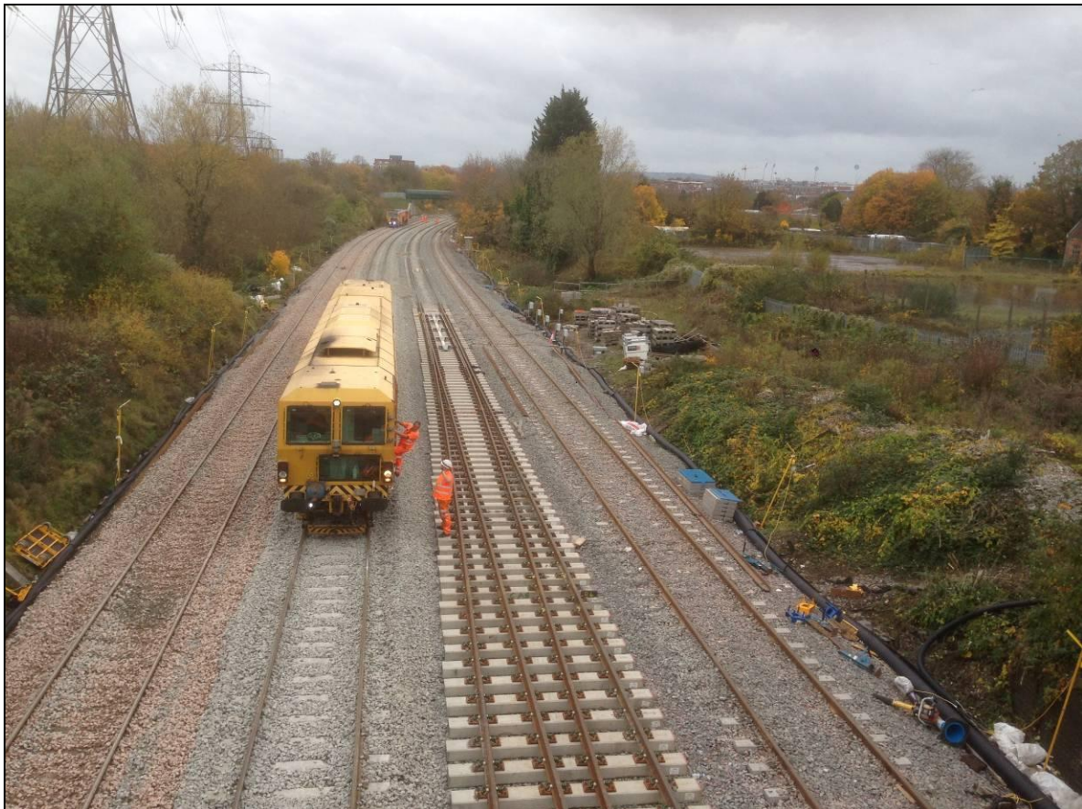
Looking north from Constable Road when works nearly completed (9/11/18)
