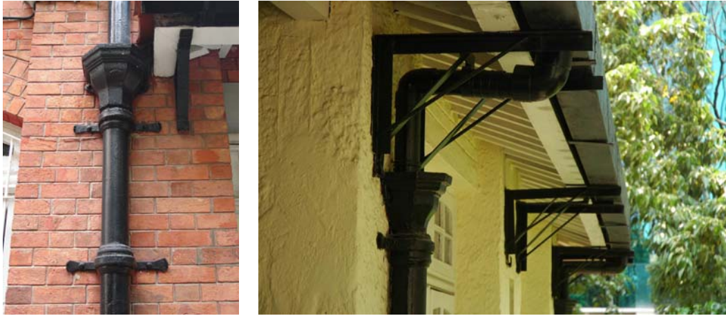
Fig. 481. Existing cast iron downpipes with hopper head of earlier period.
