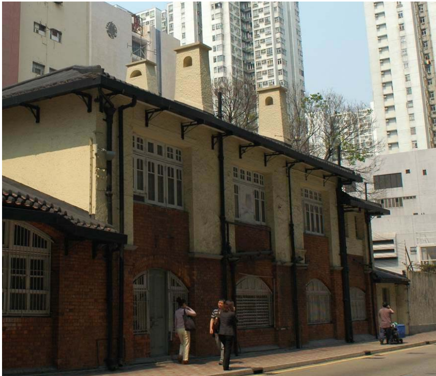
Fig. 480. Multiple roof forms finished with double-layered pan and rendered roll tiles.
