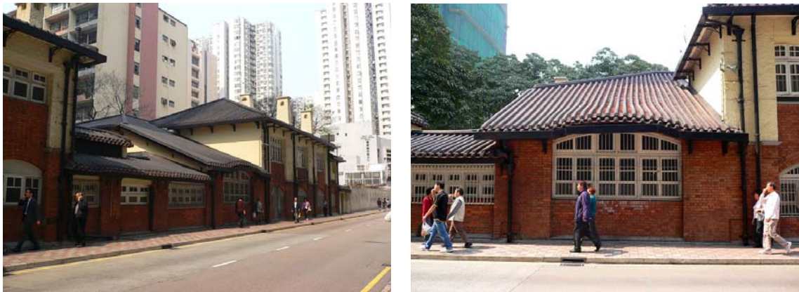
Fig. 444. The multiple roof forms supported by brackets
