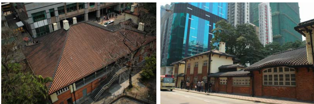
Fig. 479. Multiple roof forms finished with double-layered pan and rendered roll tiles.
