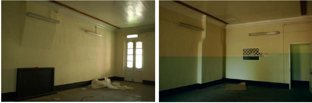
Fig. 459. Blocked fireplace at 1/F main building.
