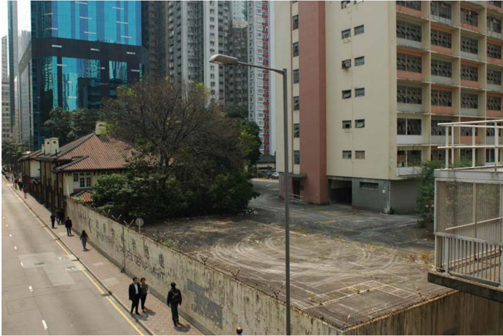
Fig. 468. The present boundary wall facing Electric Road.
