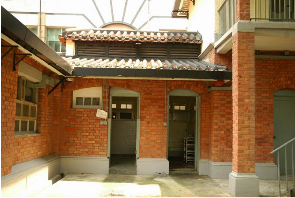
Fig. 445. Vent on top of the ridge of the pitch roof at toilet block.
