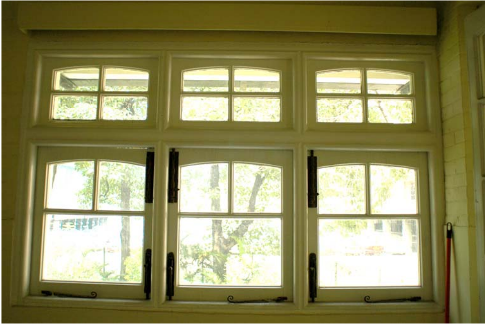
Fig. 454. Segmental-headed window with copper ironmongery.
