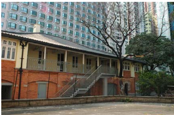
Fig. 447. The front façade with distinctive unfinished red brickwall and creamy white roughcast wall finishes
