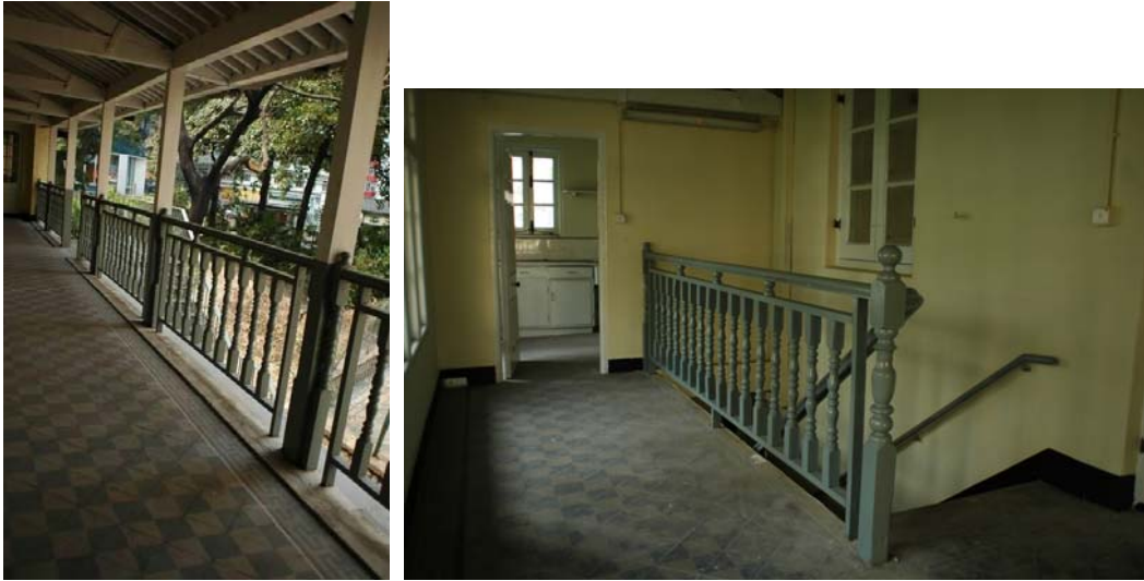
Fig. 456. Encaustic floor tiles at 1/F of main building.
