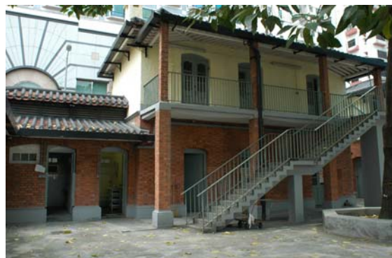
Fig. 447. The front façade with distinctive unfinished red brickwall and creamy white roughcast wall finishes
