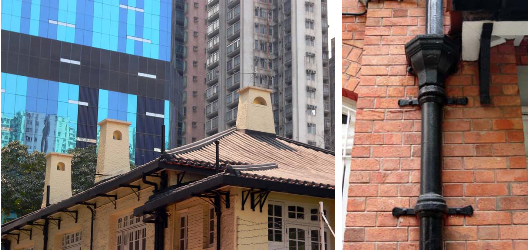
Fig. 448. Prominent chimney and downpipes at the main building
