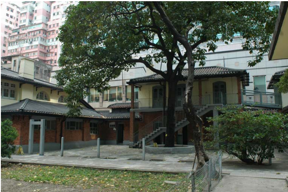
Fig. 466. The mature tree in the courtyard between Annex A and B.
