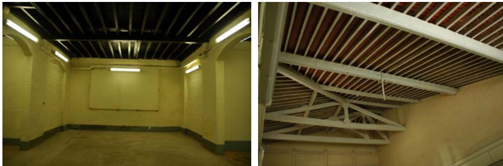
Fig. 477. Timber floor and roof structures
