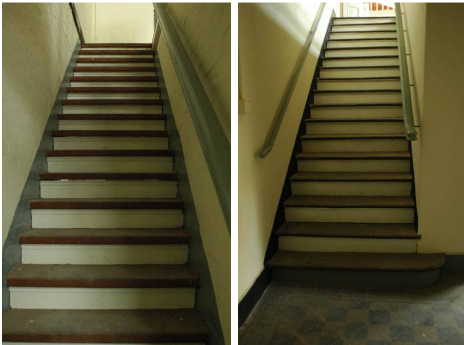
Fig. 453. Two internal timber staircases.
