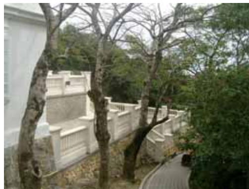
10. Recent Construction of Terraces
