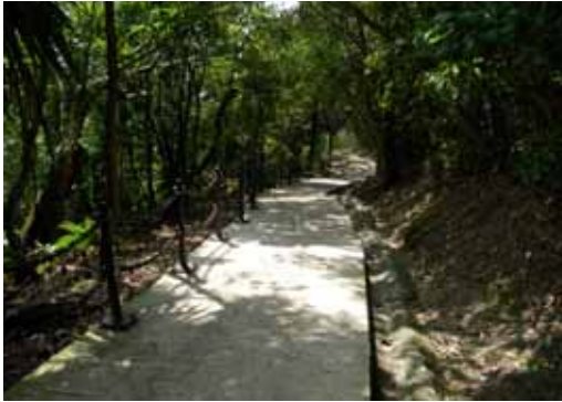
19. Part of Governor's Walk (concreted)
