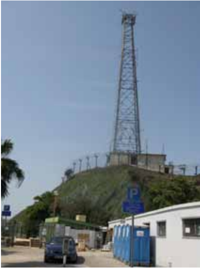
Photo of Radio Tower (Source : Oval Feb 2009)
