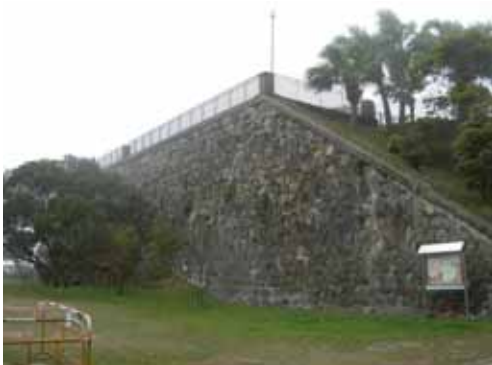
11. Whole view of the retaining wall
