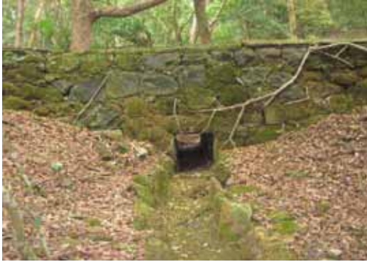
15. Stone retaining wall
