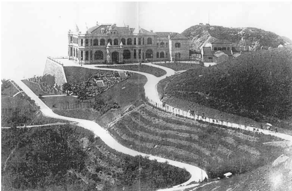
4. View of Mountain Lodge circa 1903 showing slope planting between and below the access roads with apparent new tree planting on upper slopes. (Courtesy of Public Records Office)
