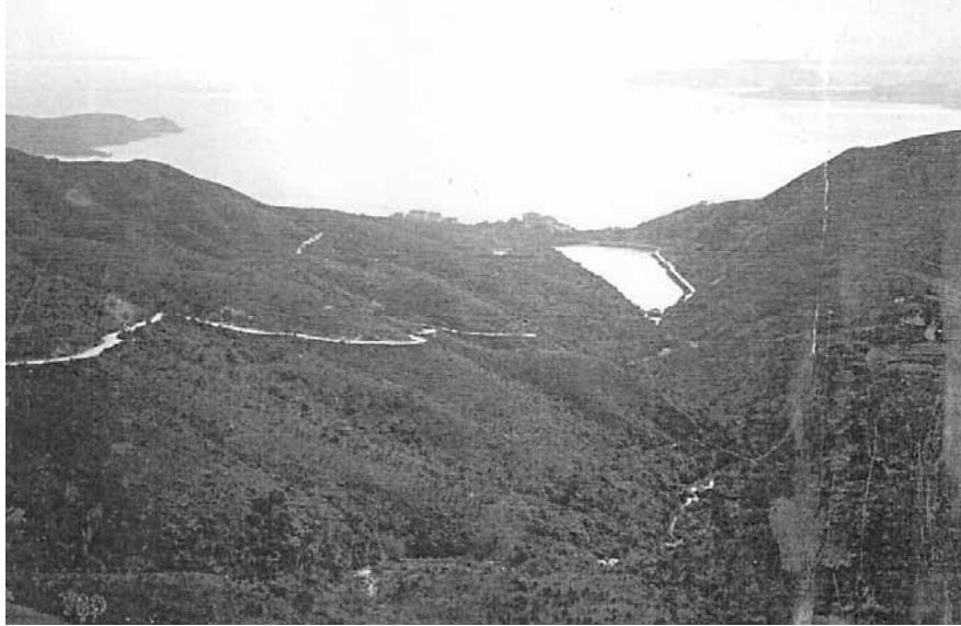
2. View of Pokfulam Reservoir (built 1863) from the Peak (late 1800s). Tree planting on the surrounding slopes was necessary to protect the reservoir from soil erosion. (Courtesy of the Public Records Office)
