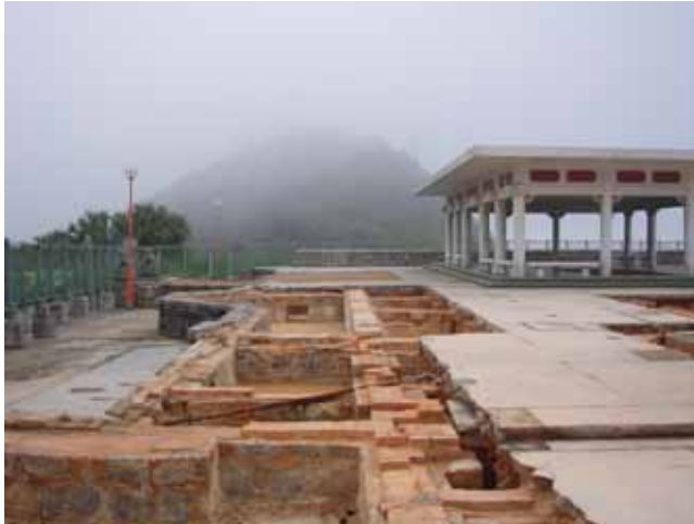
Photo of Foundation of Former Mountain Lodge (FML) (Source : Oval Feb 2009)
