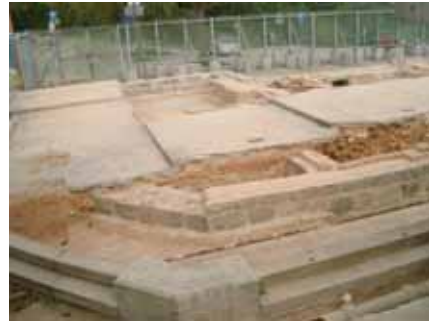
8. Exposed FML foundations under archaeological investigation in February 2009
