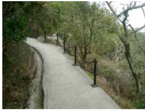
18. Railing work commencing
