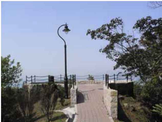
Photo of Circular Viewing Platform (Source : Oval Feb 2009)
