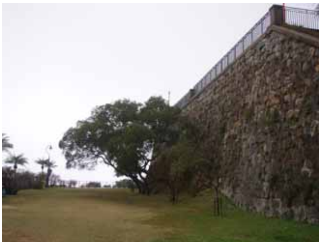
Photo of Retaining wall in Victoria Peak Garden (Source : Oval Feb 2009)
