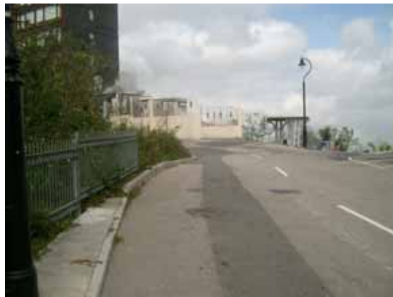
2. Disappearing sidewalk at Mount Austin Road
