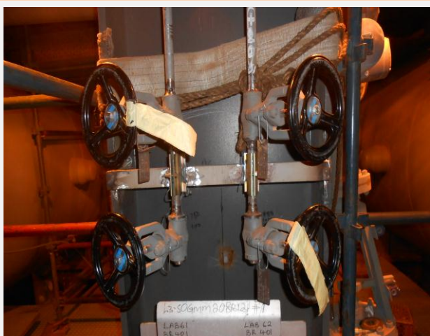
Work started on the installation of drains on various systems
