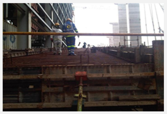
Course ash conveyor ready for concrete pour on 1 December
