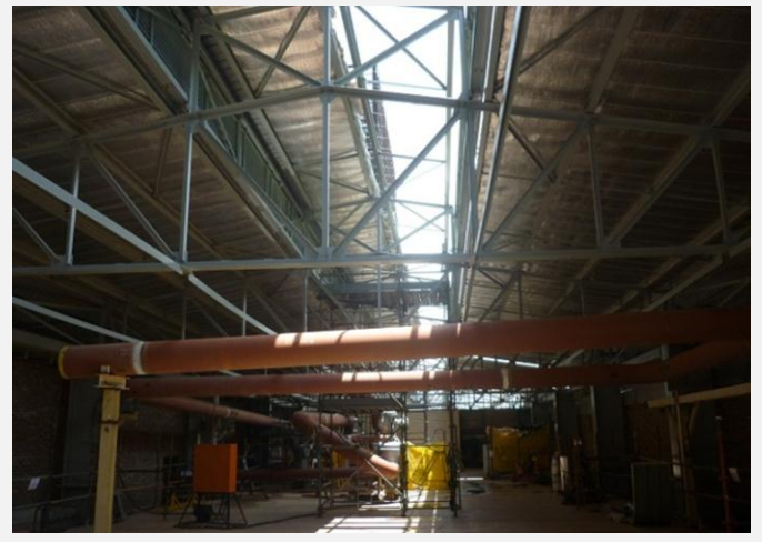
Aux bay roof cladding progressing well
