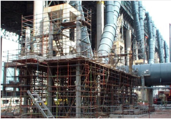
CPP building top floor columns construction in progress
