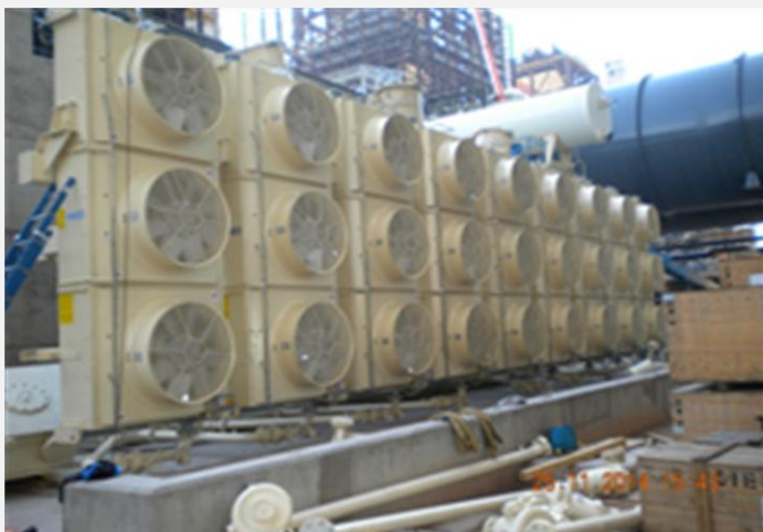
Generator transformer ancillary installation is progressing well
