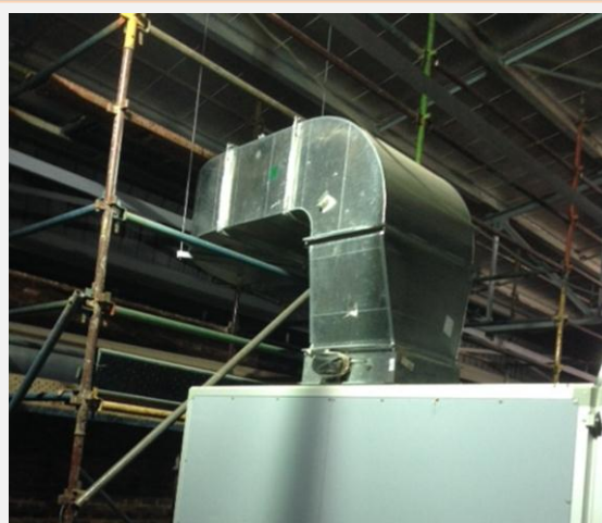
HVAC Plant room: duct installation resumed this week
