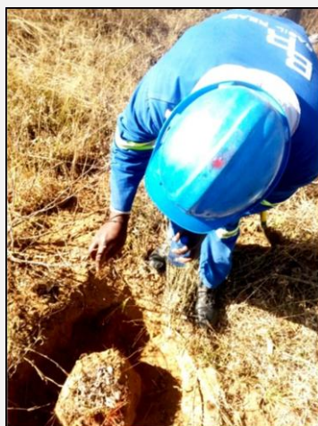
Digging very carefully!
