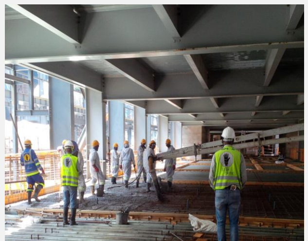
Re-bar installation progressing well on Unit 2- 13.6m level
