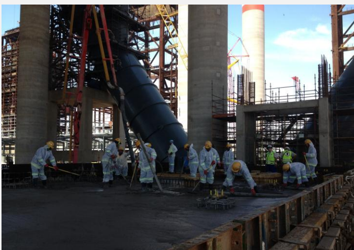
The 15M level of the ACCCT building is cast on Unit 1
