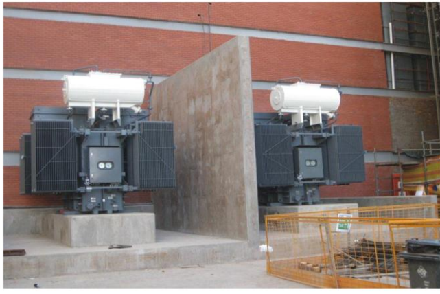
Both Service Transformers installed and auxiliaries assembled on Unit 4
