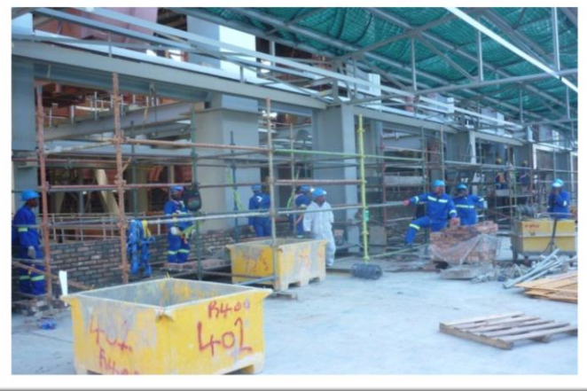
20.6 m level slab completed. External brick work has begun on Unit 3
