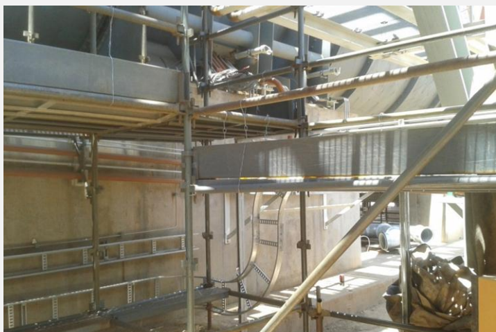
Access to Unit 5 ID Fans
