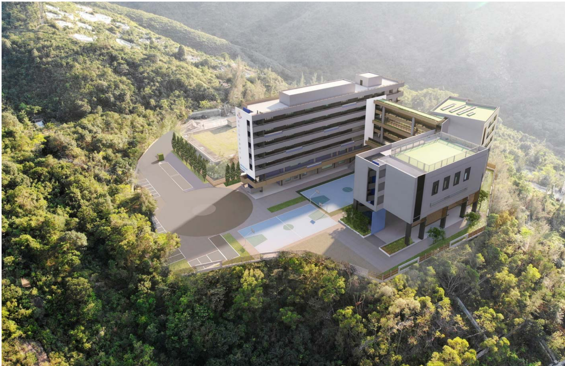
從東北面望向小學的構思透視圖 PERSPECTIVE VIEW OF THE PRIMARY SCHOOL FROM NORTHEAST DIRECTION
