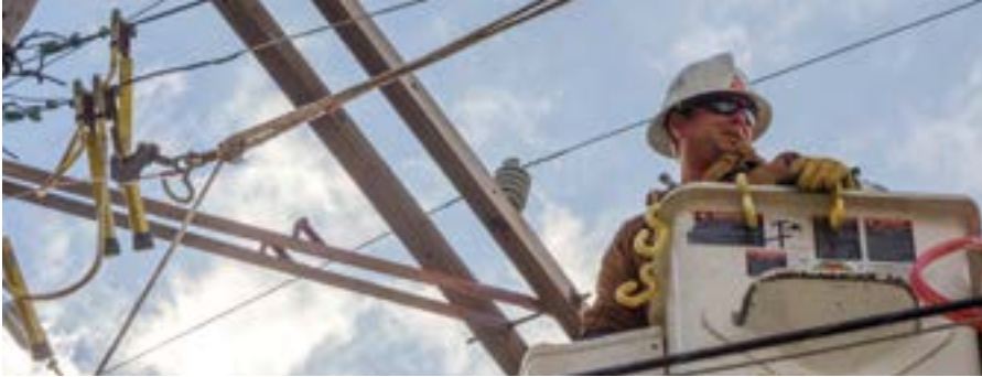
Power Restoration in New Jersey [Source: Liz Roll, FEMA 11/2/2012]
