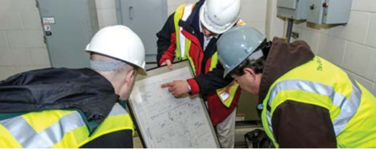
Engineers plan repair of Bay Park Waste Water Treatment Plant damaged by the storm surge from Hurricane Sandy.[Source: K.C. Wiley, FEMA. 03/20/2014]
