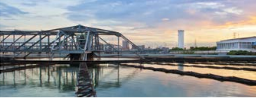
Water Treatment Plant
