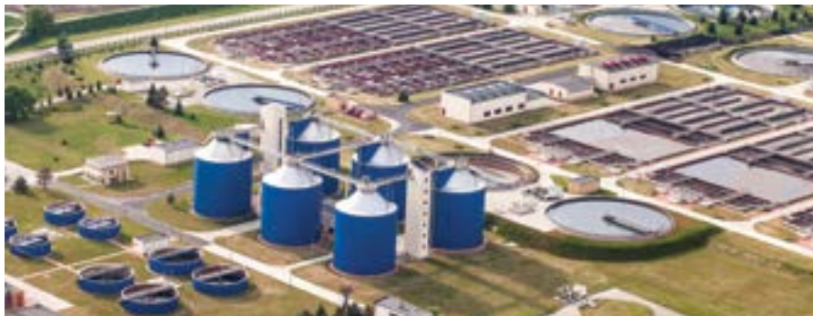
Aerial View of a Sewage Treatment Plant
