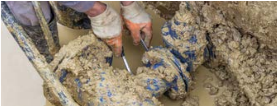
Utility worker fixing broken watermain
