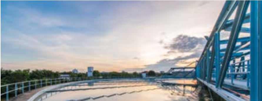
Settling Tank at Water Plant
