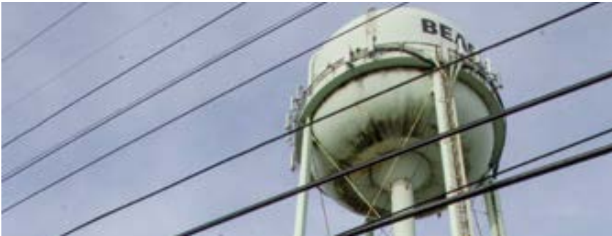
The water treatment plant in Beach Haven, N.J. being run by U.S. Army Corps of Engineer generators three weeks after Hurricane Sandy hit. [Source: Liz Roll/FEMA. 11/20/2012]
