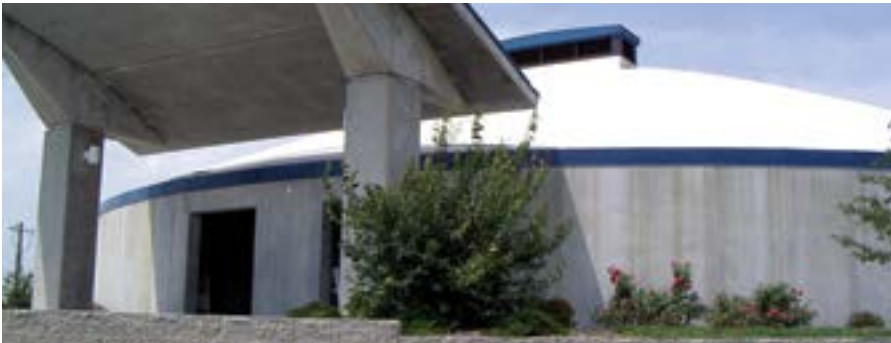
This tornado shelter for 400 campers at the Iowa State Fairgrounds outside Des Moines, IA. When not in use as an emergency shelter, the large multi-purpose building is used by both the fairground sta and campers for restrooms, showers, a laundry area, o ces, and meeting space. [Source: FEMA. 07/24/2004]
