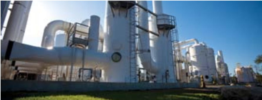
Fuel shortages will pose significant challenges for the water sector.
