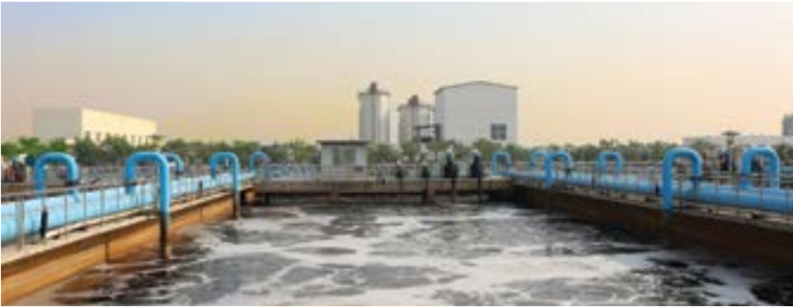
Activated Sludge Process for Sewage Treatment
