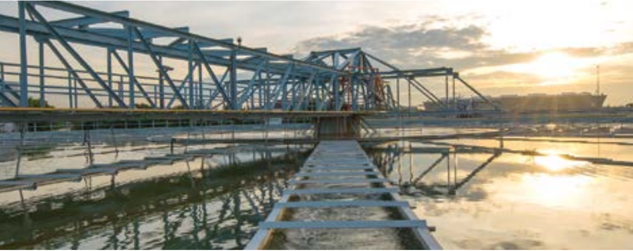
Water Purification Plant
