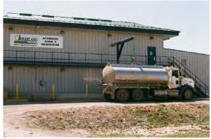
Reservoir that is located east of Provincial Highway 60 and south of Acheson Road, has capacity for 4,000 cubic metres of storage. The County operates one truck fill station which is located at the Acheson Zone 3 Reservoir. There is one dedicated pump for this truck fill station. Both reservoirs comply with storage volume requirements (including fire requirements) identified in Alberta Environment Standards and Guidelines for Municipal Waterworks and Storm Drain Systems (2006).
