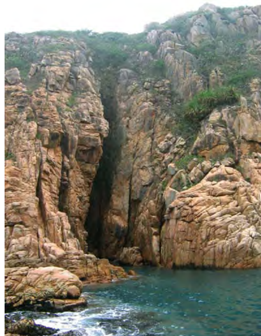
Vertical cracks at Tai Tau Chau
