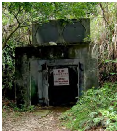
Portal of the 240 m tunnel
