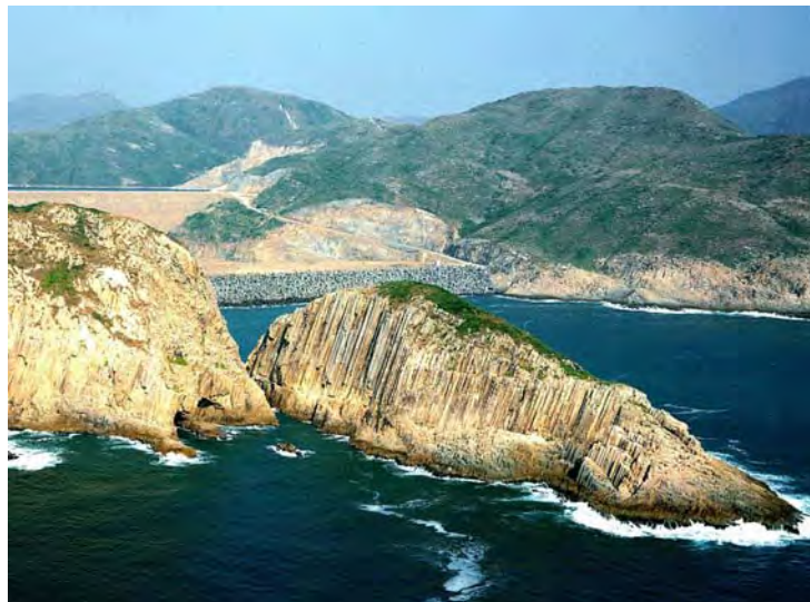
The East Dam of High Island Reservoir from Po Pin Chau
