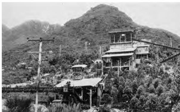
Portal of the 110m main ore haulage tunnel
