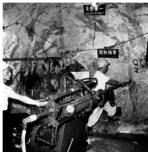
Blasthole drilling in the mining tunnel
