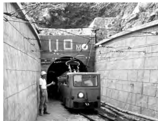
Portal of the 110m main ore haulage tunnel
