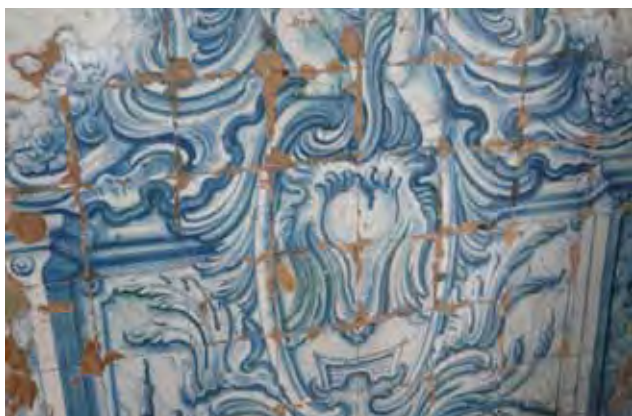
Fig. 7. Glaze damage on Portuguese tiles situated within the convent (Photo: Perside Omeda).
