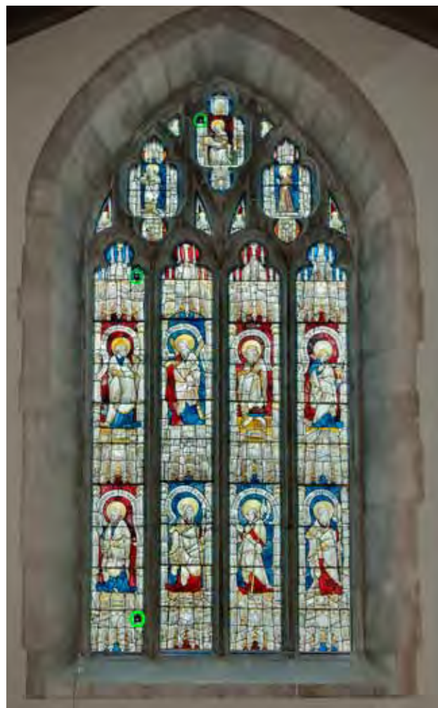
Fig. 1. Window with Apostles, the Pietá, and other Saints in 2011 after treatment and re-installation. MFA 25.213.1-.21, Maria Antoinette Evans Fund. A wire at the sill connects a datalogger probe in the interspace; glass sensors for monitoring are circled in green (Photo © Museum of Fine Arts, Boston, 2013).
