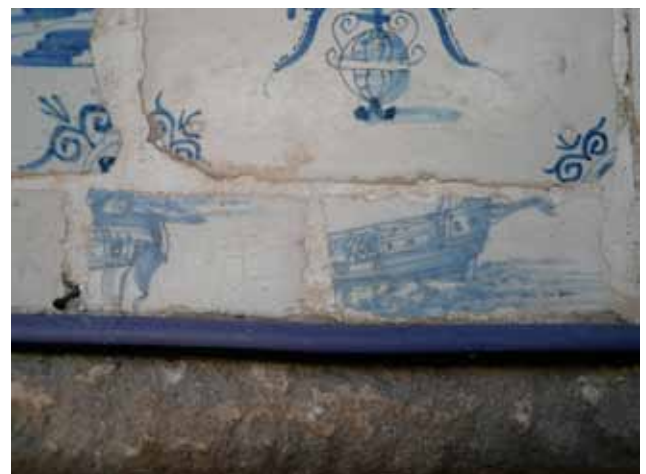
Fig. 4. Tiles 'cut down' to fit the remaining space in the niche (Photo: Kate van Lookeren Campagne).
