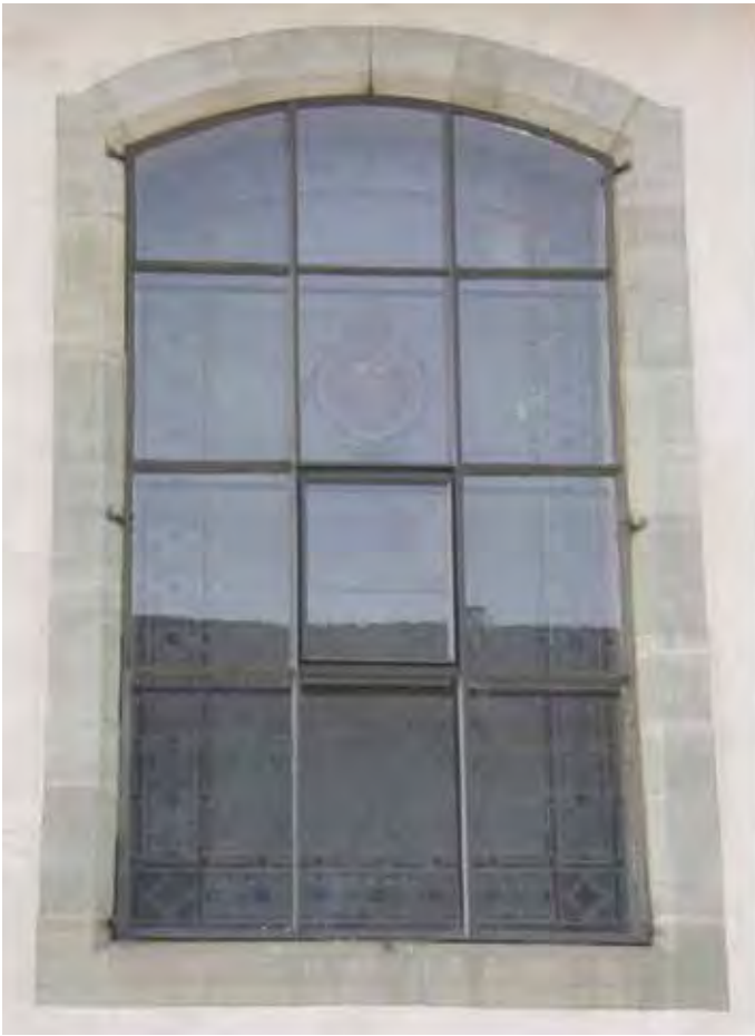
Fig. 1. Unventilated protective glazing fitted in a metal or wood frame: 'Église des Capucins' in Romont, installed around 1950 (left); Parish church of Frauenfeld-Oberkirch, installed probably before or around 1900 (right). Photos: authors.
