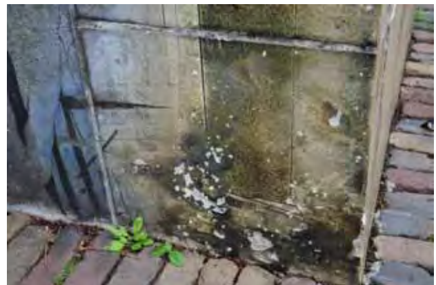
Fig. 2. Detail of ‘Ripped Archive Box’ showing the damage to the ceramic (Photo: R. Morelissen).
