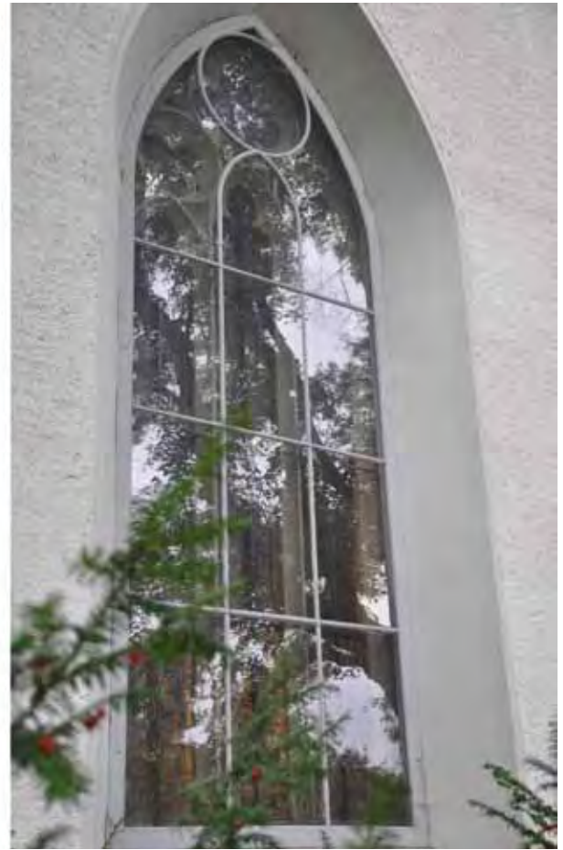
Fig. 1. Unventilated protective glazing fitted in a metal or wood frame: 'Église des Capucins' in Romont, installed around 1950 (left); Parish church of Frauenfeld-Oberkirch, installed probably before or around 1900 (right). Photos: authors.
