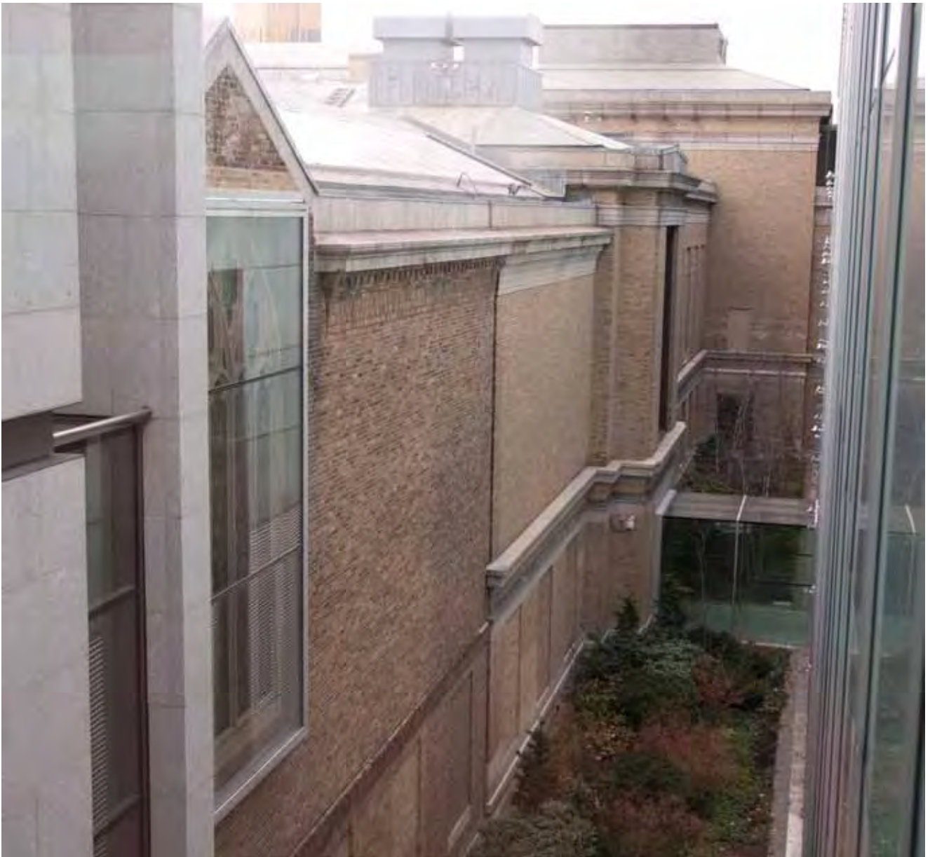
Fig. 4. Exterior view with IGU covering (Photo © Museum of Fine Arts, Boston, 2013).
