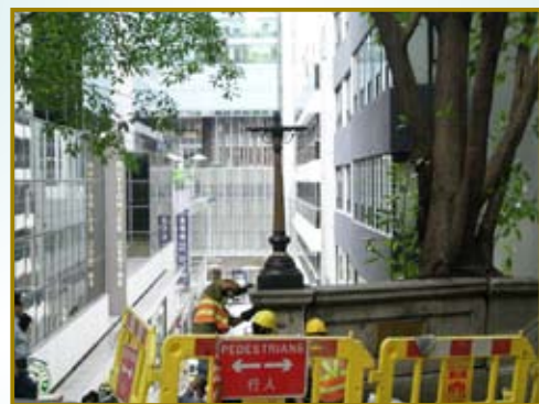
Resetting the gas lamp and stone column to vertical
