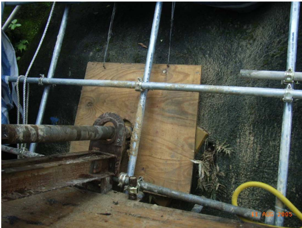
Photo 2 - A plywood should be placed and mounted above the sponge to fix the sponge in place
