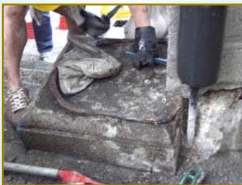
Clearing the tree roots from the foundation of stone column
