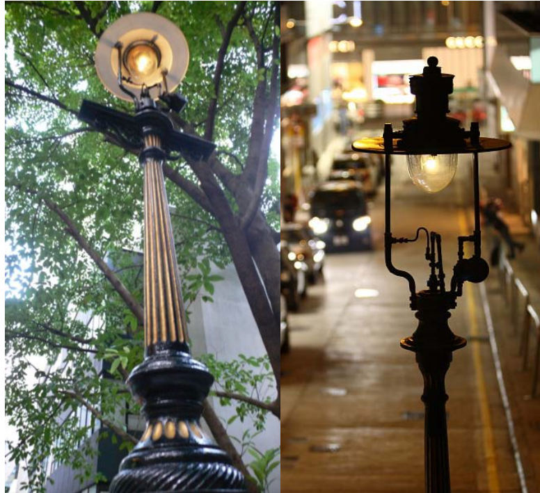
Photo 2.2 – The existing gas lamps surmounting at the crest and toe of the stone steps
