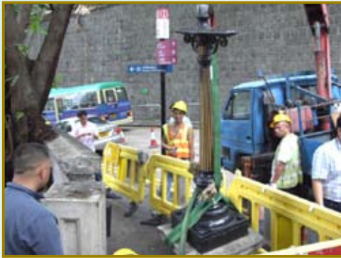
Lifting up the tilted gas lamp for the repair work
