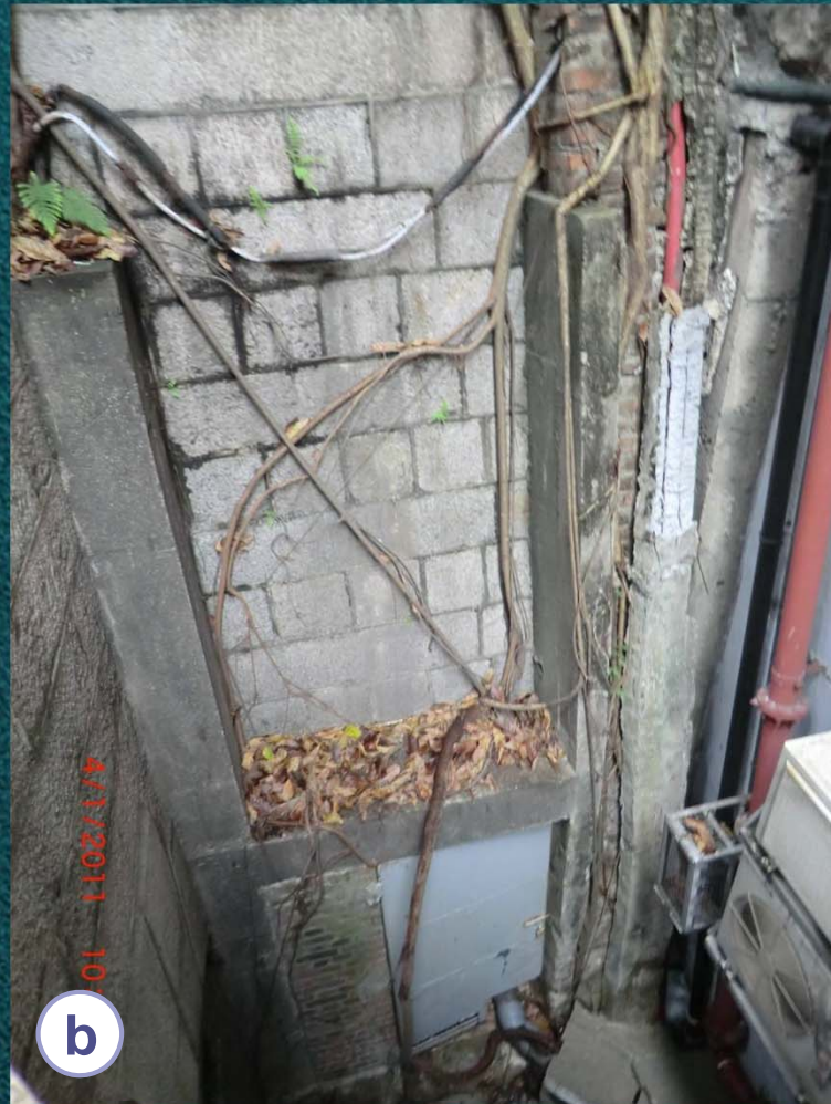
Before slope upgrading works
