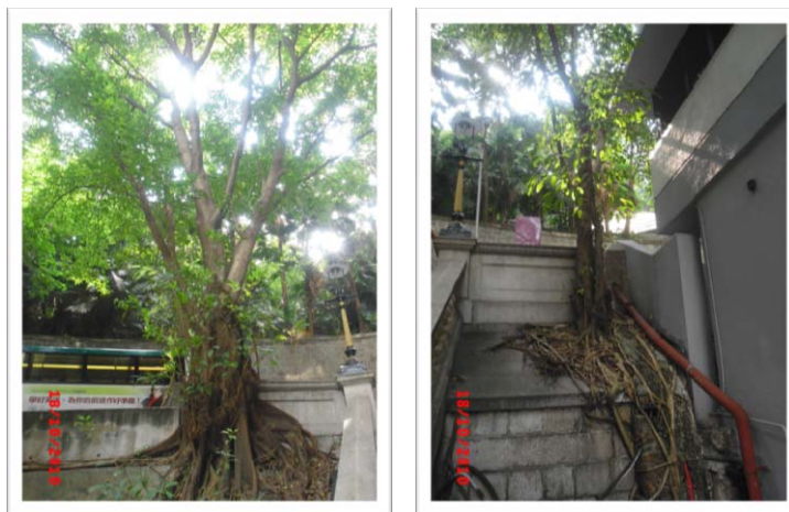
Photos 4.3 and 4.4 – Existing wall trees located above Portals 43 and 44.
