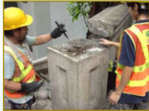
Clearing the surface of stone column for resetting the gas lamp
