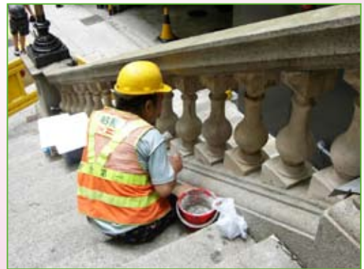
Specialist contractor repairing the damaged balustrades
