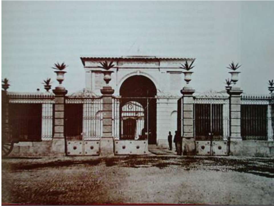
Figure 2-9. Dos de Mayo Hospital (Under construction)
