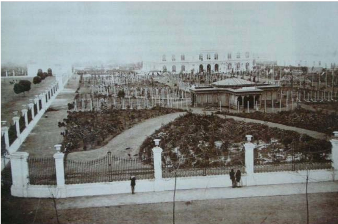
Figure 3-7. Exposition Compound under construction, 1871.
