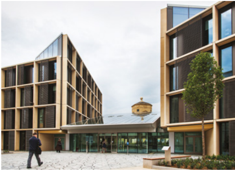
Above: The final paving in front of the main entrance Right: The tiles being carefully laid outside the building Below: Sketch of Sir Roger Penrose's design
